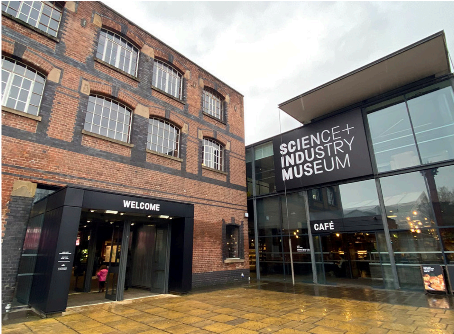
Image: External view of New Warehouse.
