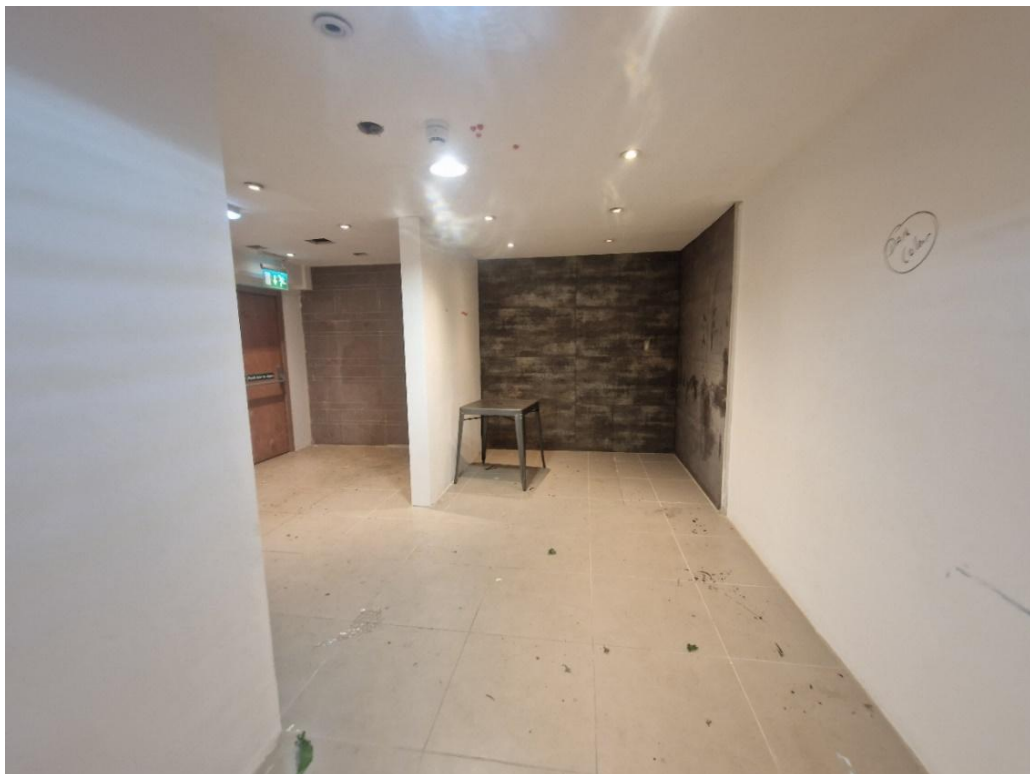
Image 8: Basement Interior view towards fire exit door, rear of unit 265
