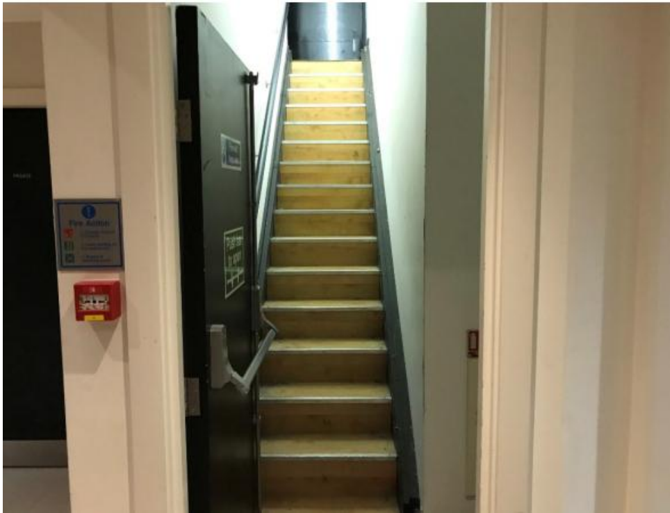
Image 9: Basement to Ground Interior view, MOE staircase to final exit onto Deansgate, this stair will serve Units 261/263 & Units 265/267
