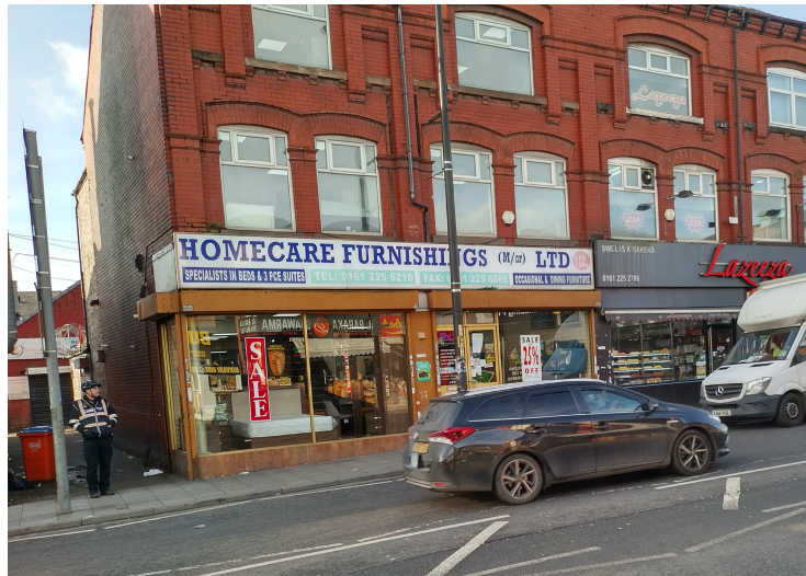
Fig.1 – Existing shop front presented to Stockport Road
