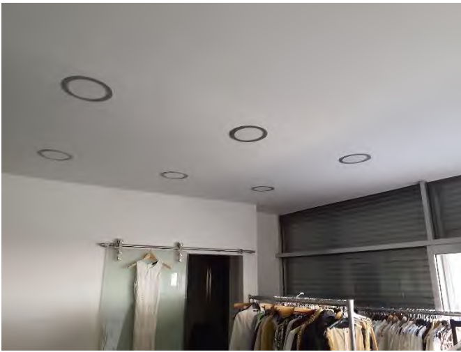
Photograph 3: Commercial unit with plastered walls and ceilings.
