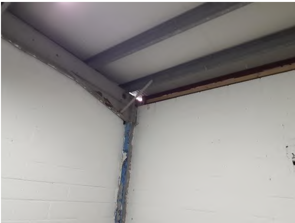
Photograph 9: Potential internal bat roost access point between the external wall and ceiling at south-eastern corner of building on Postal Street.
