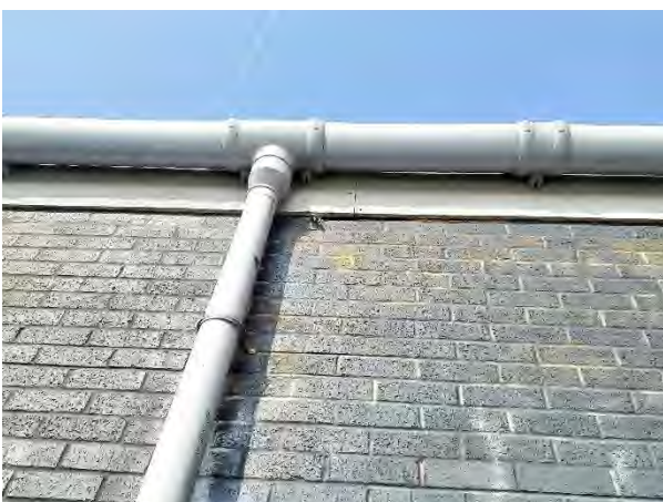
Photograph 13: External PRF along south-eastern aspect of building.
