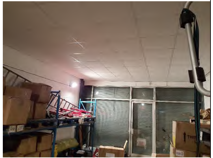
Photograph 4: Commercial unit with suspended ceilings and roof tiles.
