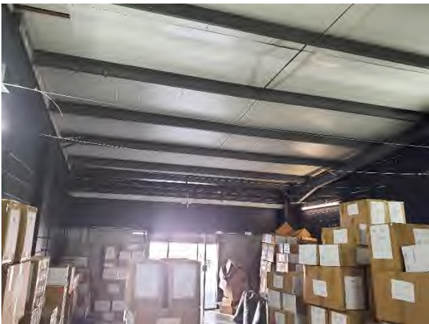
Photograph 5: Commercial unit with no internal fit-out.
