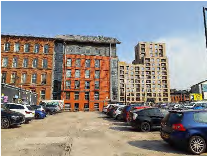
Photograph 1b: View across car park from Faraday Street looking north-east towards Postal Street.
