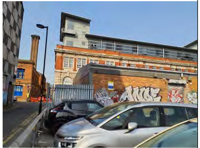
Photograph 2: Adjacent building to the north on Faraday Street.
