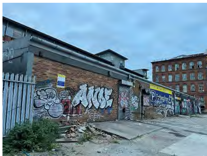
Figure 2-2: Building view of surveyor 2 positioned on south-western corner between Dean Street and Faraday Street
