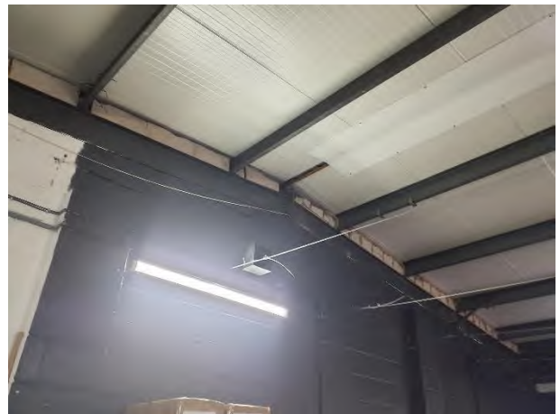
Photograph 6: Exposed steel joists along ceiling.
