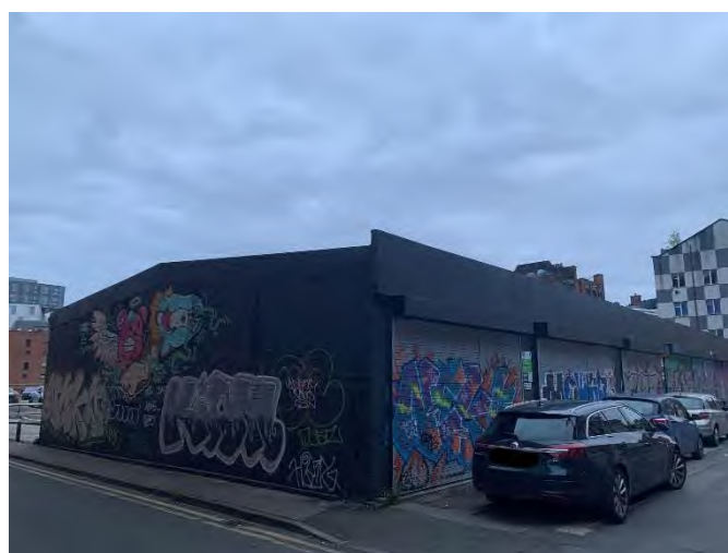
Figure 2-1: Building view of surveyor 1 positioned on north-eastern corner between Newton Street and Postal Street
