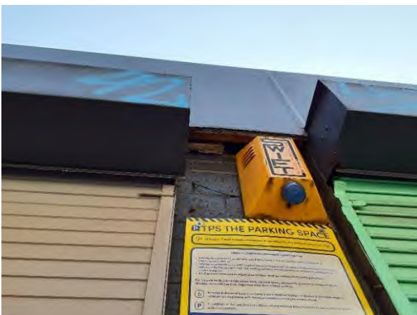
Photograph 11: External PRF on north-western aspect along Newton Street.
