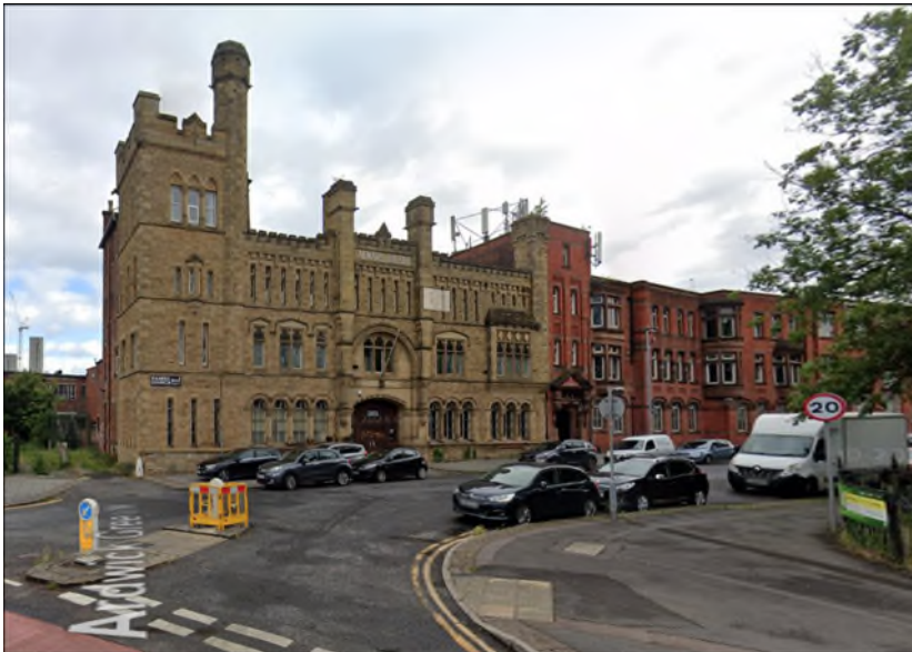
View of application building (Source: Google Maps)
