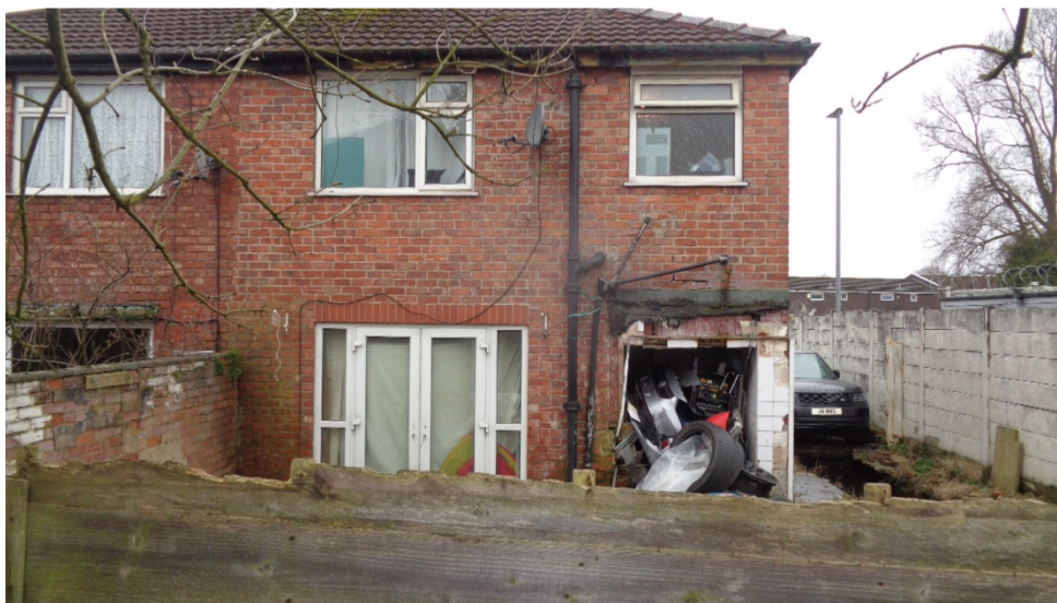
Rear Elevation of application property.
