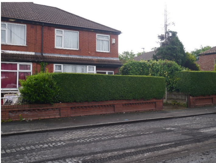
Front Elevation of adjacent property. Nr 301
