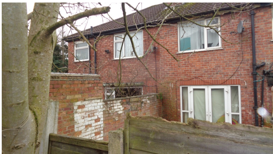
Rear Elevation of application property.
