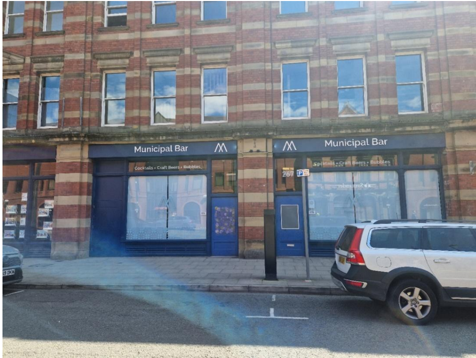
Image 1: Present Shopfront Elevation, Deansgate, Manchester
