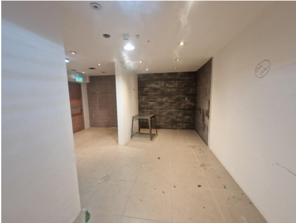
Image 9: Present Ground Floor Interior view, rear of unit 265
