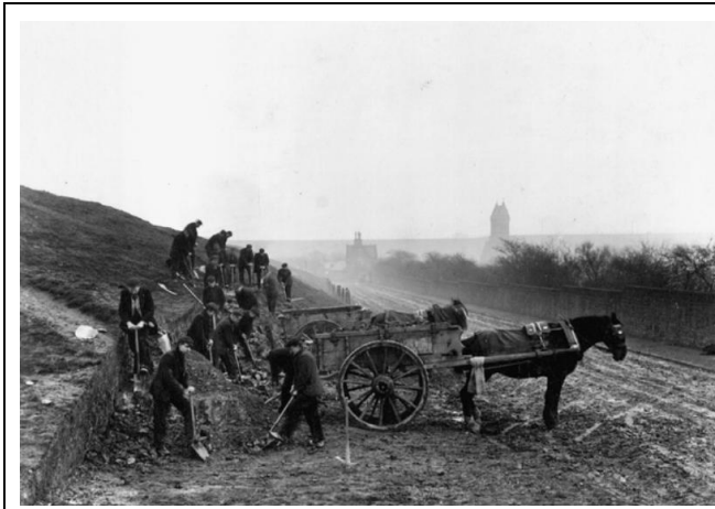
Figure 11: Infrastructure works on Riverpark Road, formerly Cemetery Road, 1904. Source: Greater Manchester Lives.
