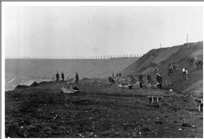
Figure 12: Infrastructure works within the Site, 1904. Source: Greater Manchester Lives.
