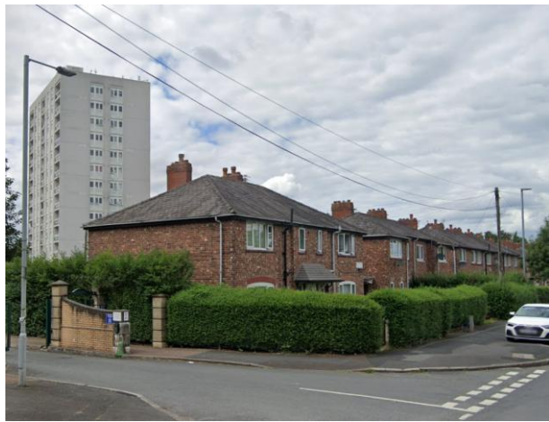
Figure 48: Tower blocks and low scale housing in TCA 3A.
