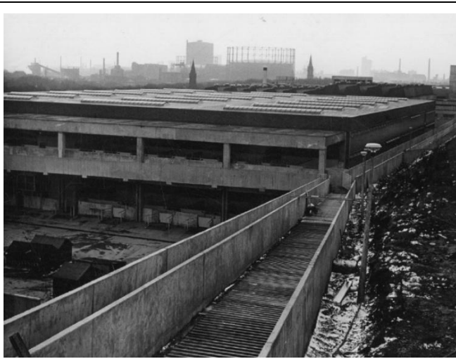
Figure 22: Cattle ramp from rail sidings to lairage, 1965.
