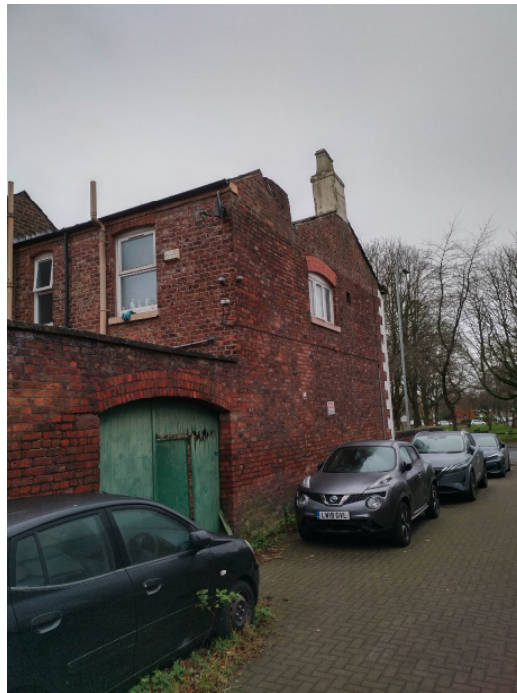
Fig.2 – views of the front and rear of 161 Slade Lane
