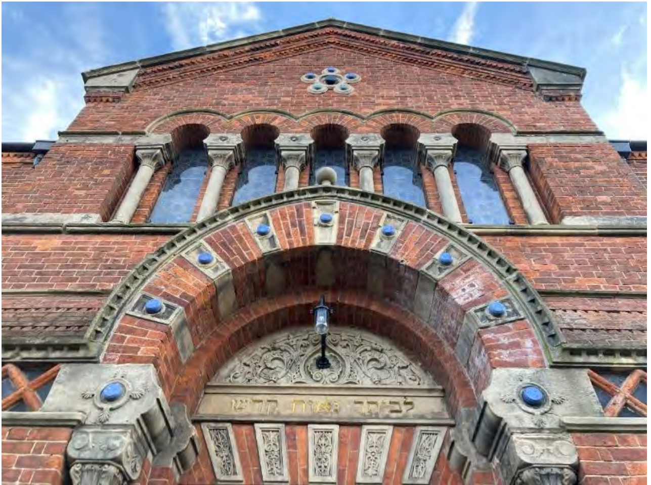
Figure 4.5 – detailing on the principal elevation of the synagogue
