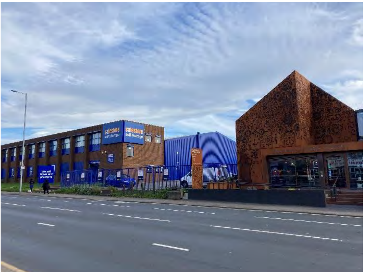
Figure 4.11 – View of the Jewish Museum and the Safestore unit on the approach along Cheetham Hill Road from the south
