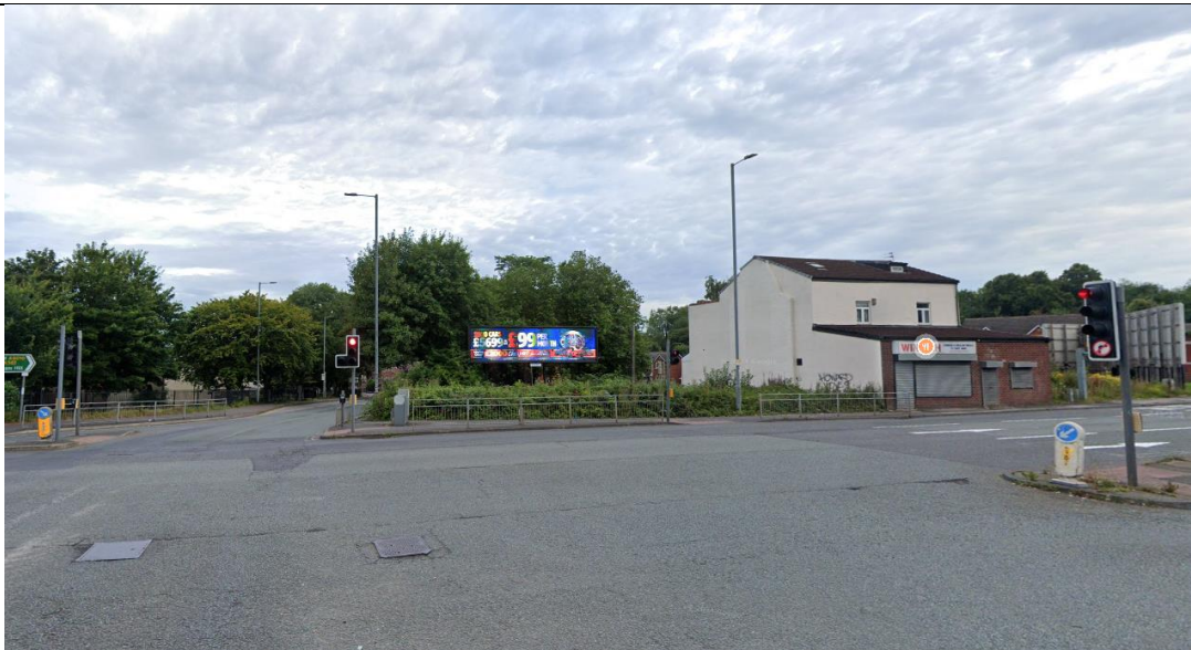
Photo 2. View towards the proposed site from Rochdale Road at the junction with Topley Street (Source: Google Maps).
