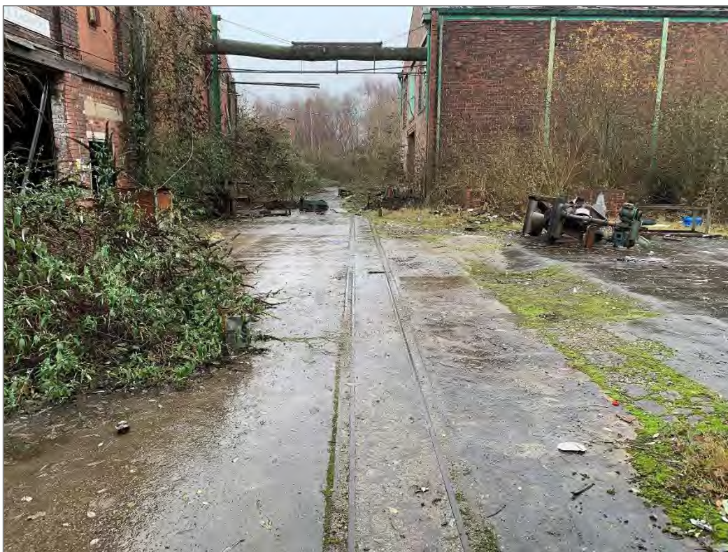
Photograph 9: 2021 Crabtree Forge. View of tramway looking east across Area 15, Area 8 building to left, Area 16 building to right
