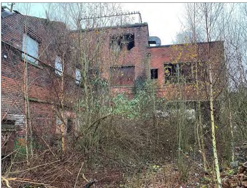
Photograph 6: Crabtree Forge. 2021 view of Area 6 and Area 4 buildings from the north of the site looking west
