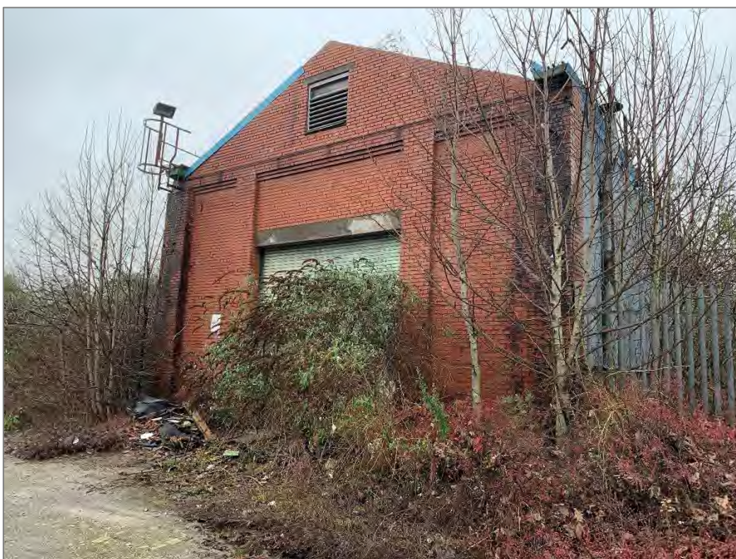
Photograph 8: Crabtree Forge. 2021 view of Area 13 building from the south of the site looking north
