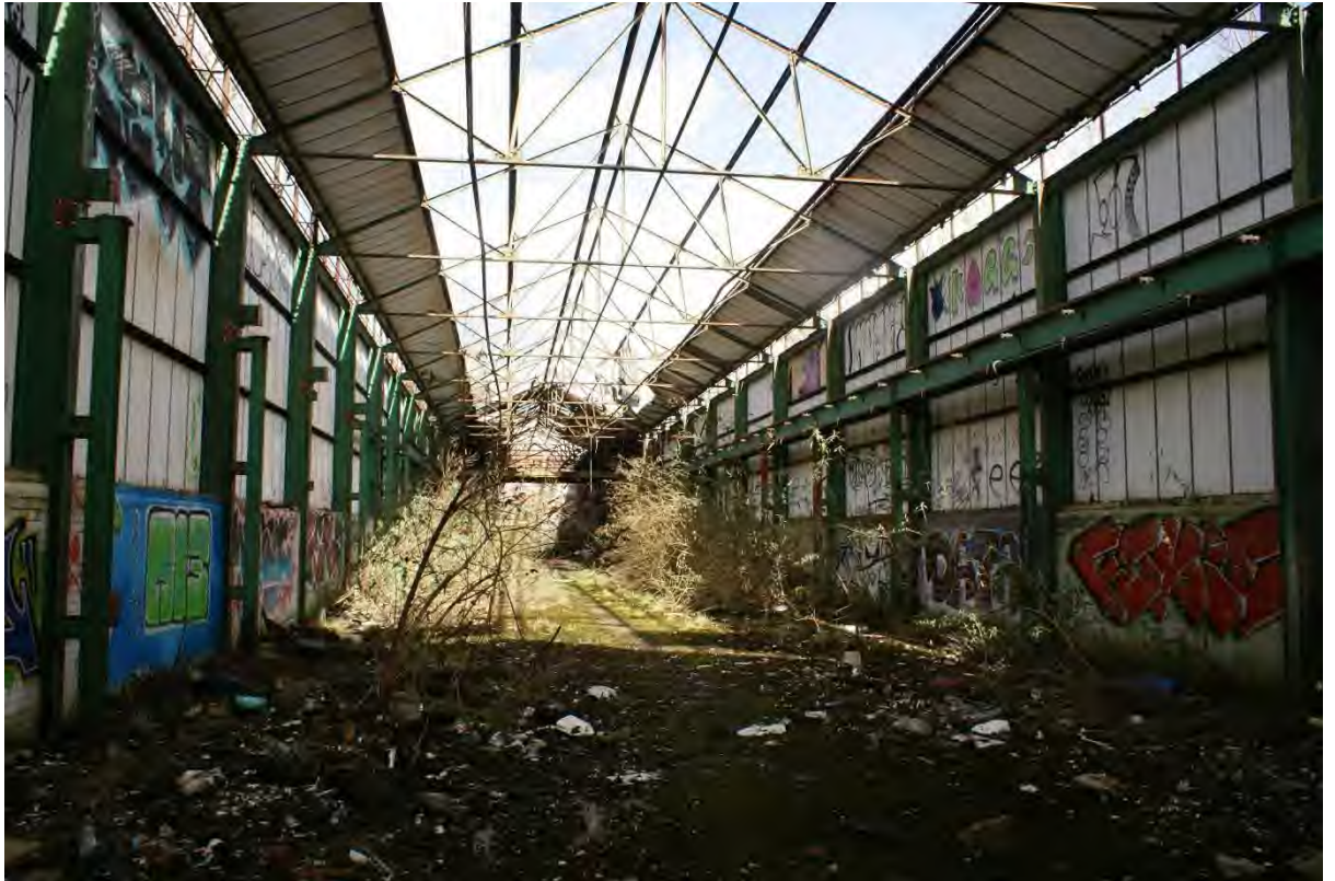
Photograph 32: Crabtree Forge 2025. Interior of Area 13 building in 2025, looking to the north
