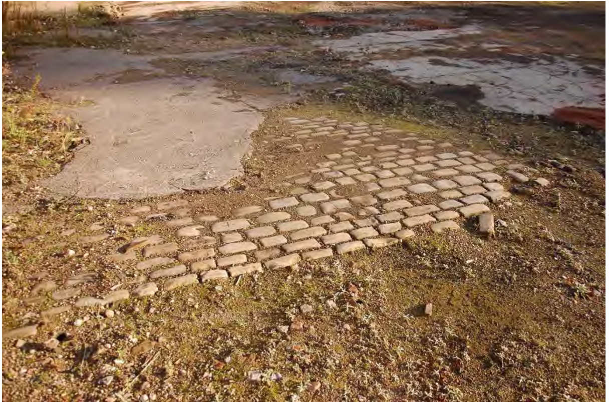
Photograph 26: Acre Works. 2024 stone sett flooring extending under later concrete surfaces – view to east
