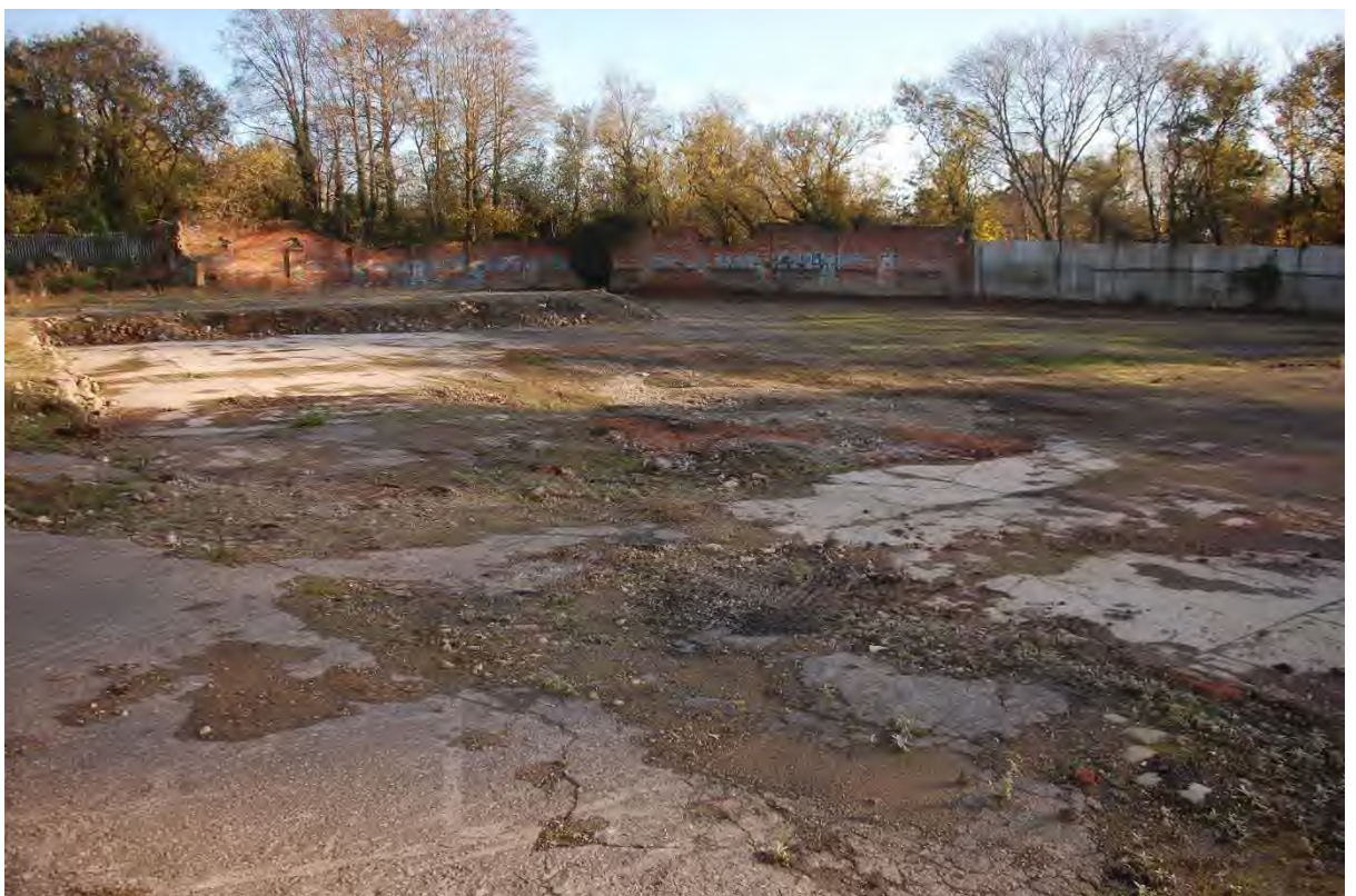
Photograph 25: Acre Works. 2024 elements of otherwise demolished buildings forming part of the south-eastern site boundary with, in the foreground and to the left, made ground and superimposed floor surfaces demonstrating the survival of the remains of different structural phases in the north-eastern part of the site - view to south east
