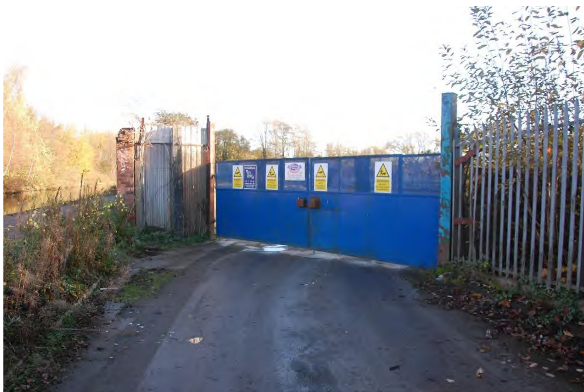
Photograph 21: Acre Works. 2024 site entrance looking east
