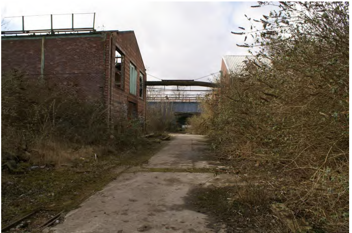
Photograph 39: Crabtree Forge 2025. View west towards Area 15, Area 16 building to left and Area 8 building to right. Tramway visible on the left.
