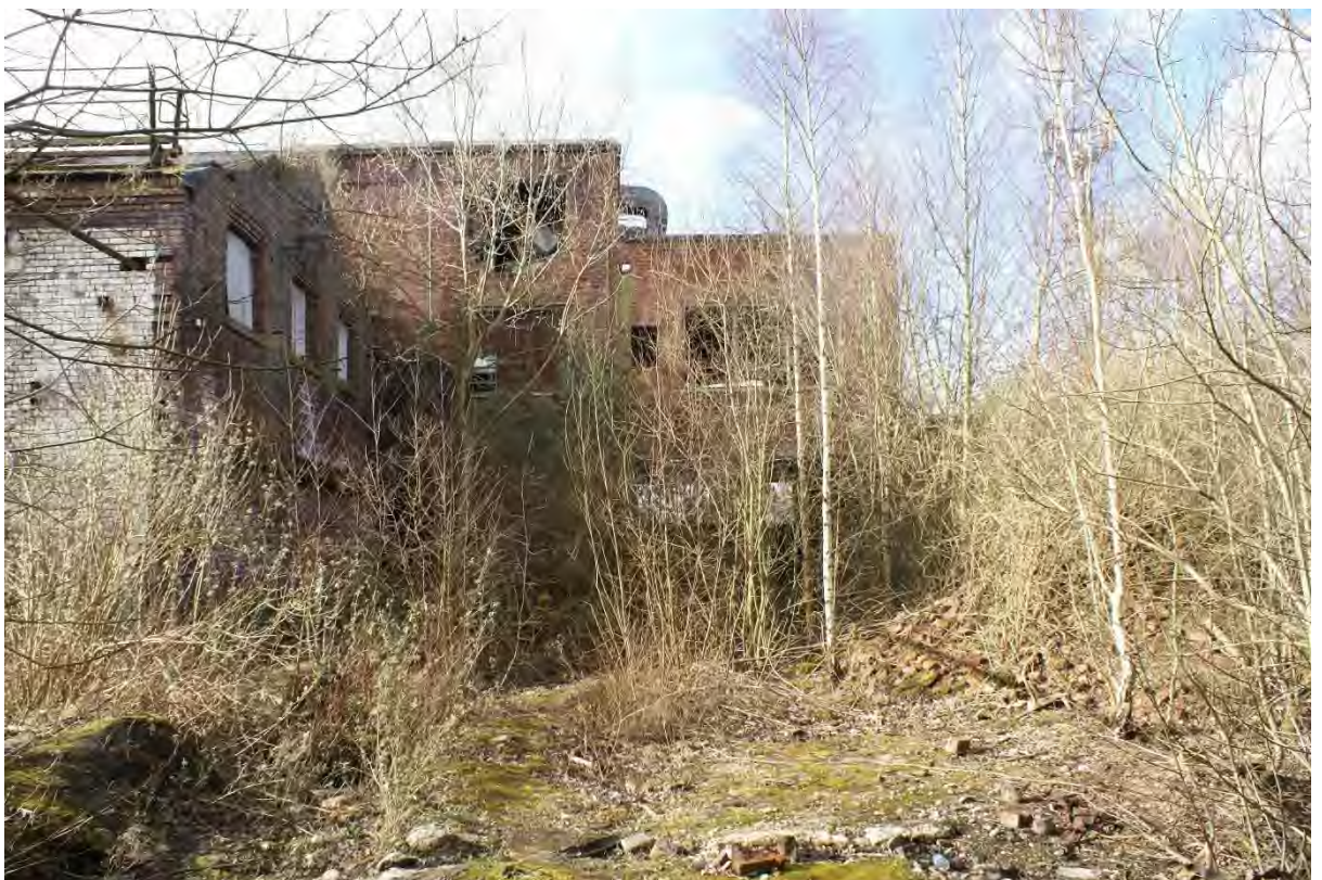
Photograph 37: Crabtree Forge 2025. View of Area 6 and Area 4 buildings from the north of the site looking west
