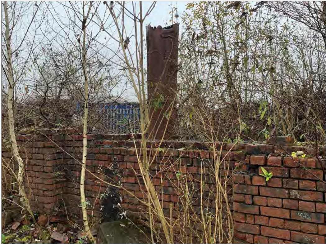
Photograph 12: Crabtree Forge. 2021 view of structure remains in the north of the site looking northeast
