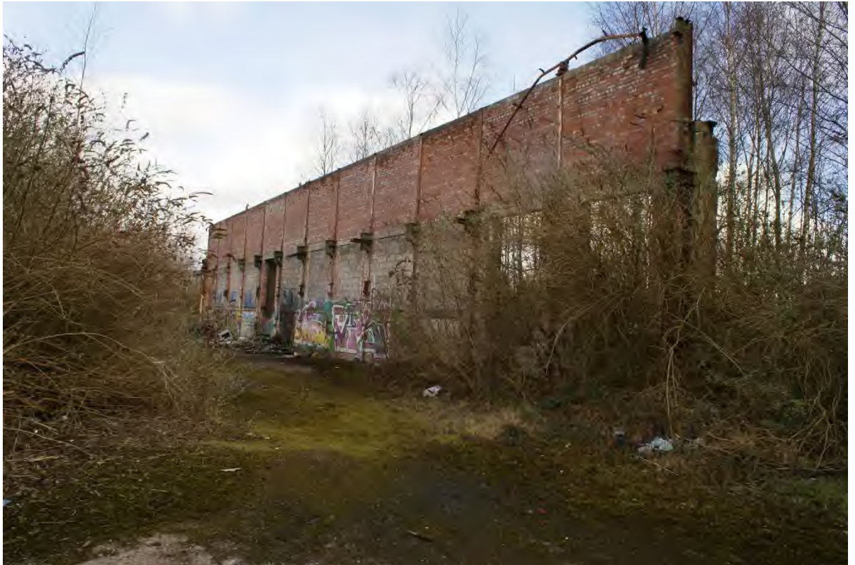
Photograph 38: Crabtree Forge 2025. East wall of otherwise demolished Area 11 building in the north-eastern part of the site. View to north east.
