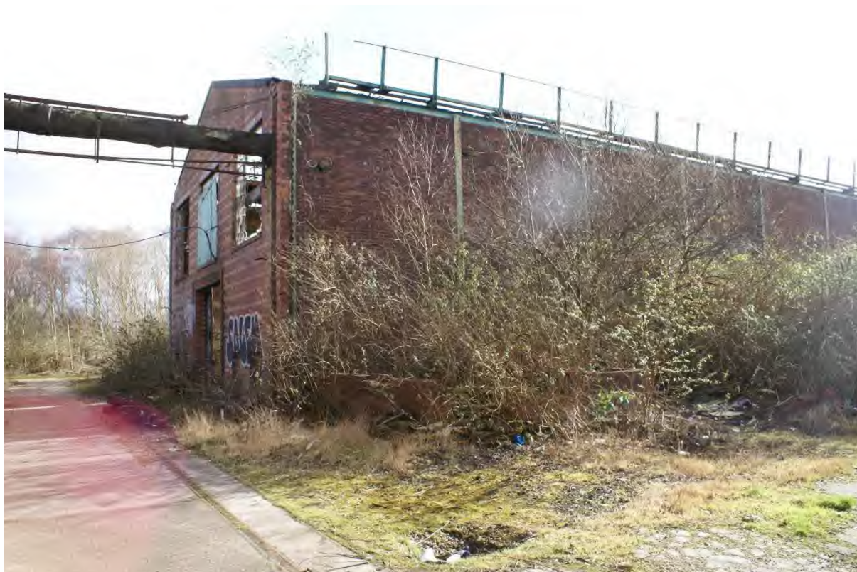
Photograph 34: Crabtree Forge 2025. View east towards the Area 6 building.
