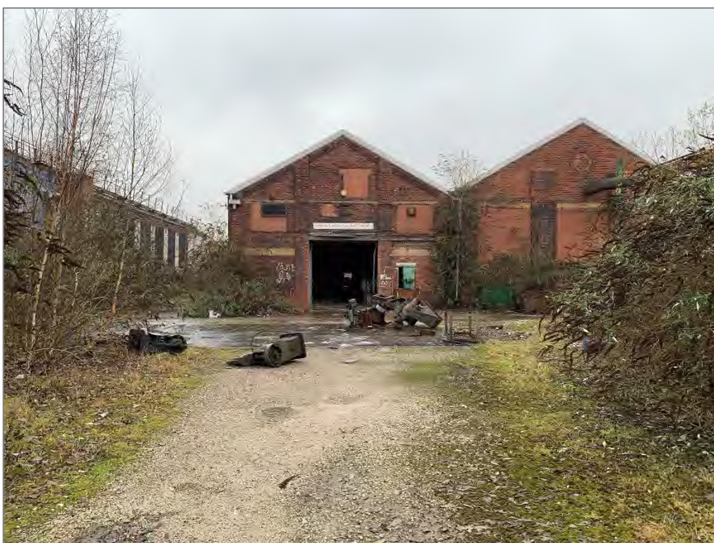
Photograph 5: Crabtree Forge. 2021 view of Area 8 buildings from centre of site looking north
