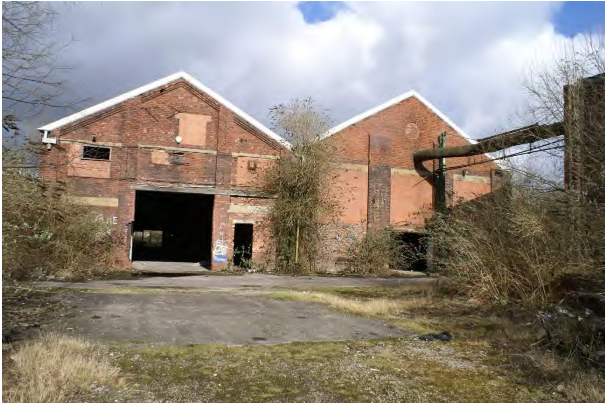
Photograph 36: Crabtree Forge 2025. View north towards the Area 8 building.
