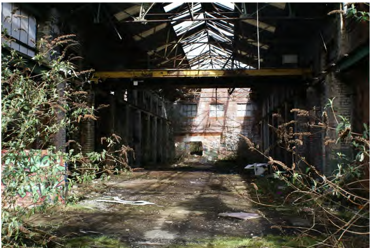
Photograph 33: Crabtree Forge 2025. Interior of the northern part of Area 6 building showing in situ overhead crane. View to north.
