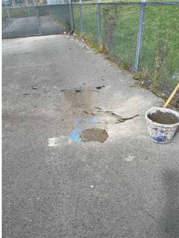
Photograph 7 WS06 following reinstatement.
