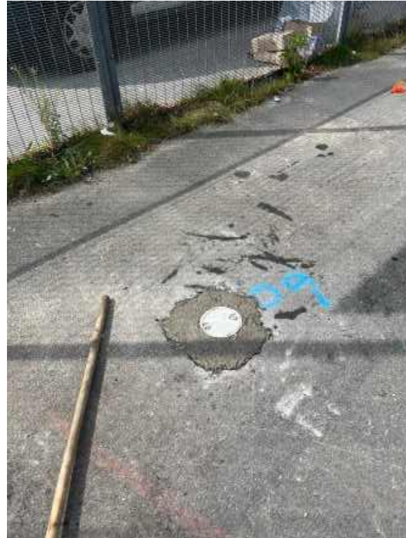
Photograph 10 WS09 following installation.
