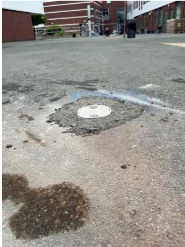
Photograph 5 WS04 following installation.
