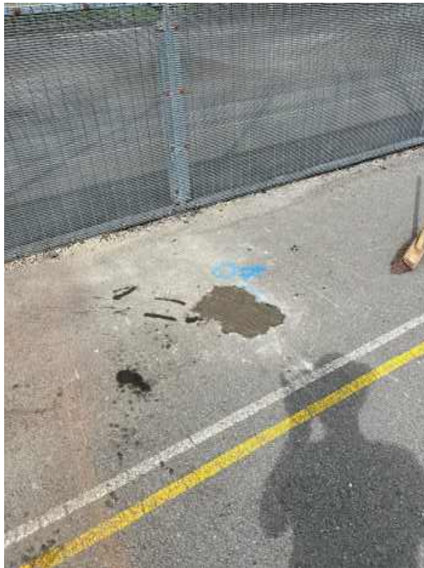
Photograph 8 WS07 following reinstatement.
