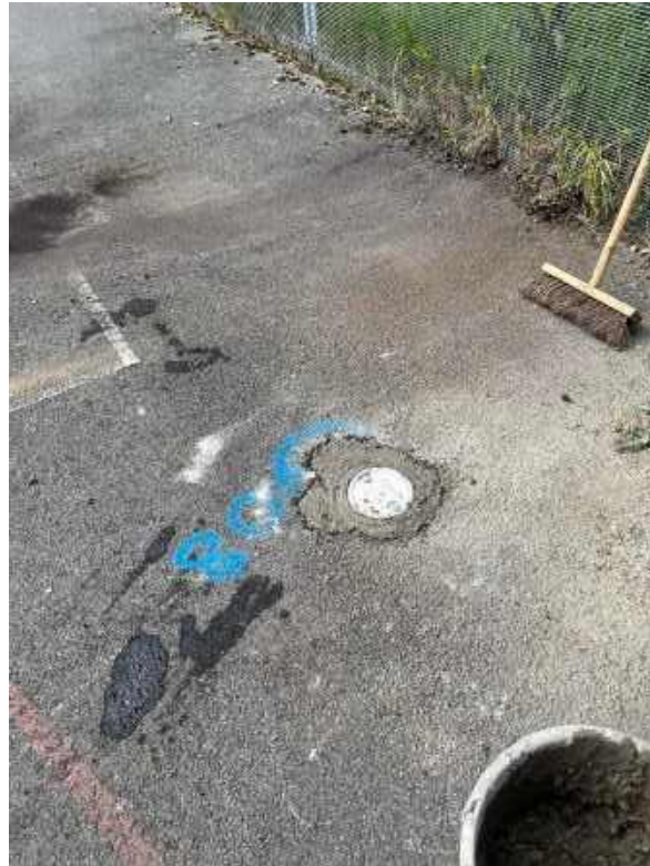
Photograph 9 WS08 following installation.
