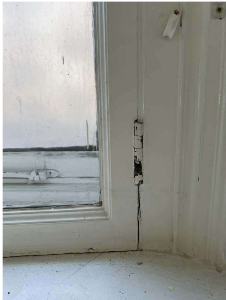
08 SECONDARY GLAZING REFERENCE 520 N/A PHOTOGRAPH EXAMPLE
