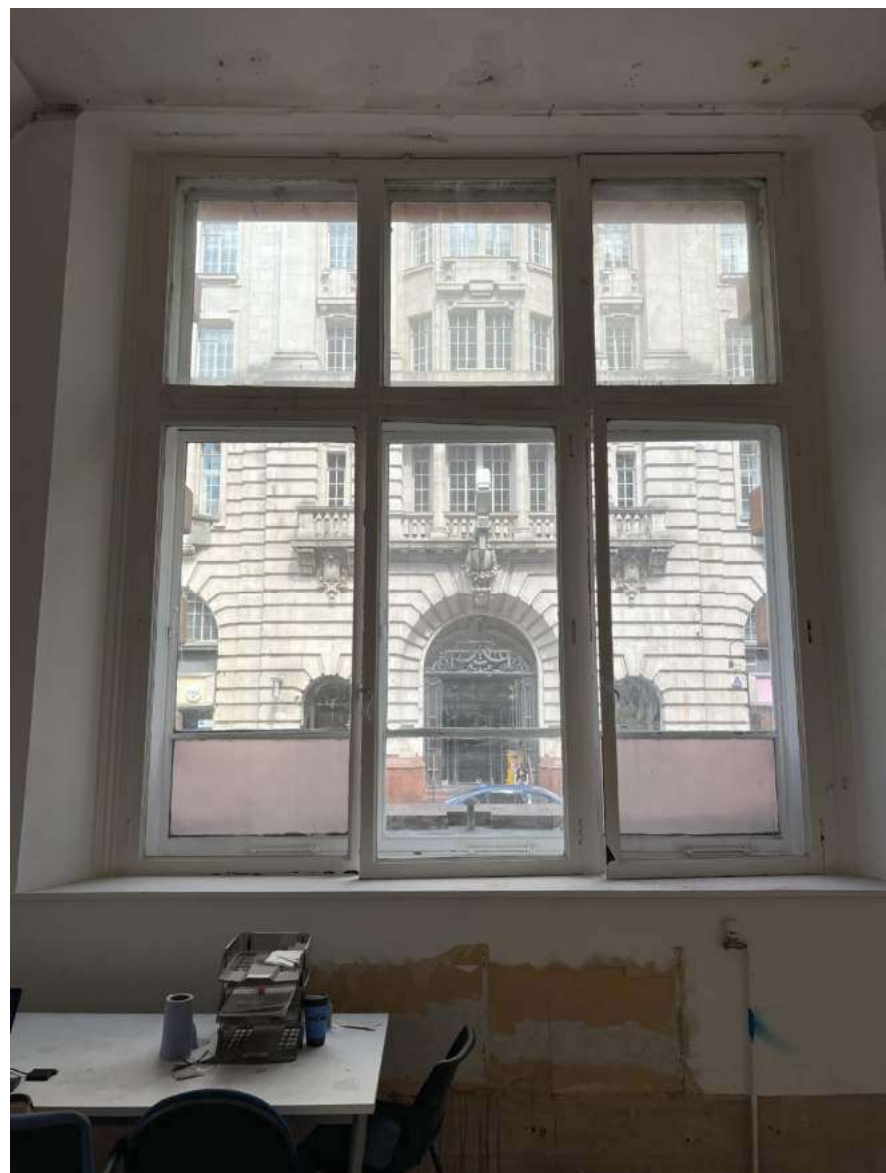
07 SECONDARY GLAZING REFERENCE 520 N/A PHOTOGRAPH EXAMPLE
