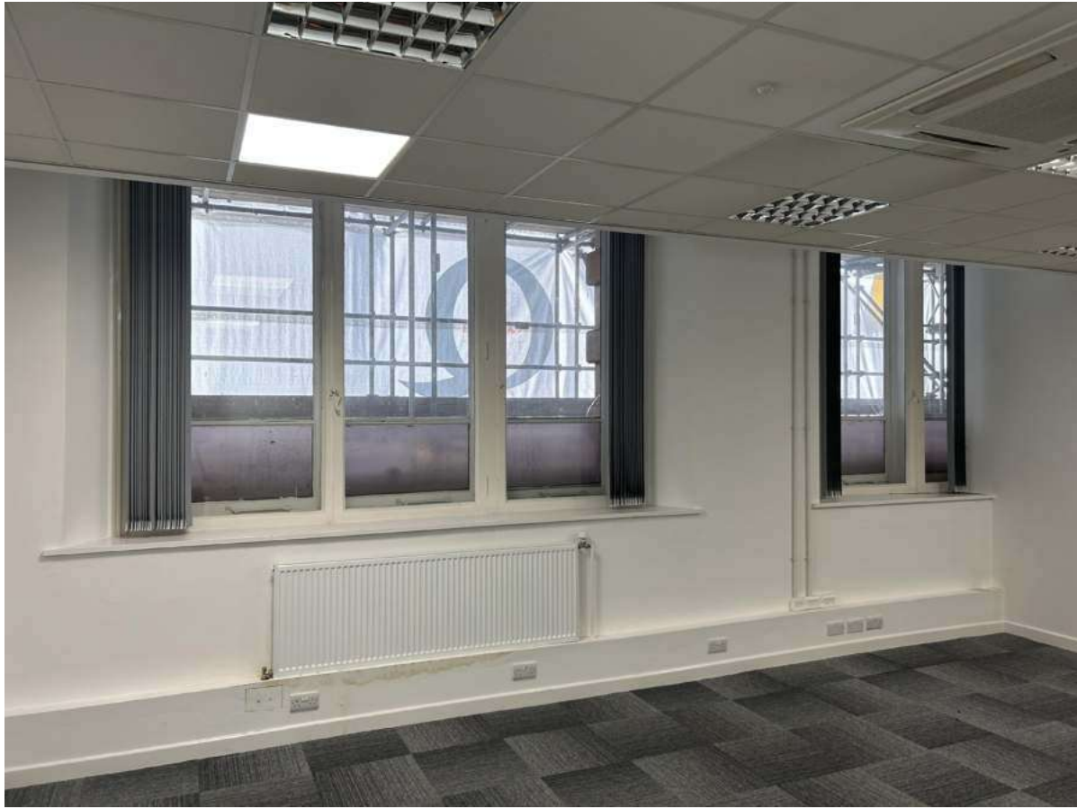
04 501 GROUND FLOOR EXISTING WINDOW 1 IMAGE NTS
