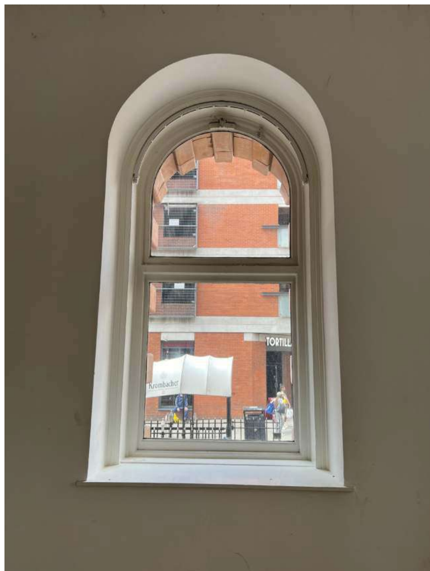
12 EXISTING PHOTOGRAPH 141 NTS EX ADJACENT WINDOW PRECEDENT
