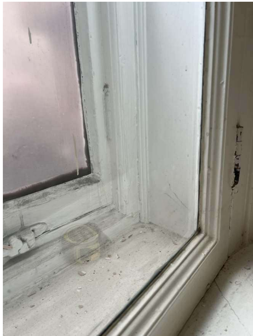
09 SECONDARY GLAZING REFERENCE 520 N/A PHOTOGRAPH EXAMPLE
