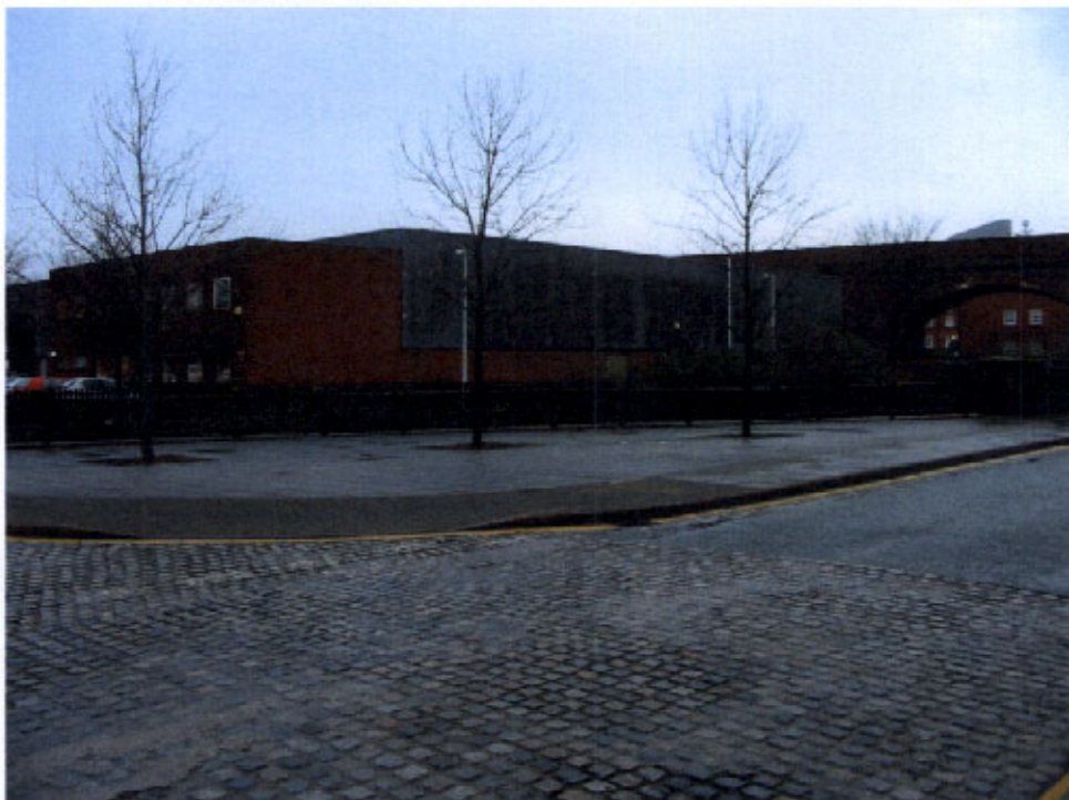
Photograph 2: View of site with Potato Wharf in the foreground and the River Medlock beyond the fencing.
