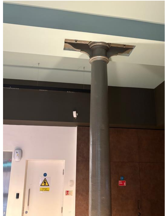
Figure 17- cast iron columns remain
