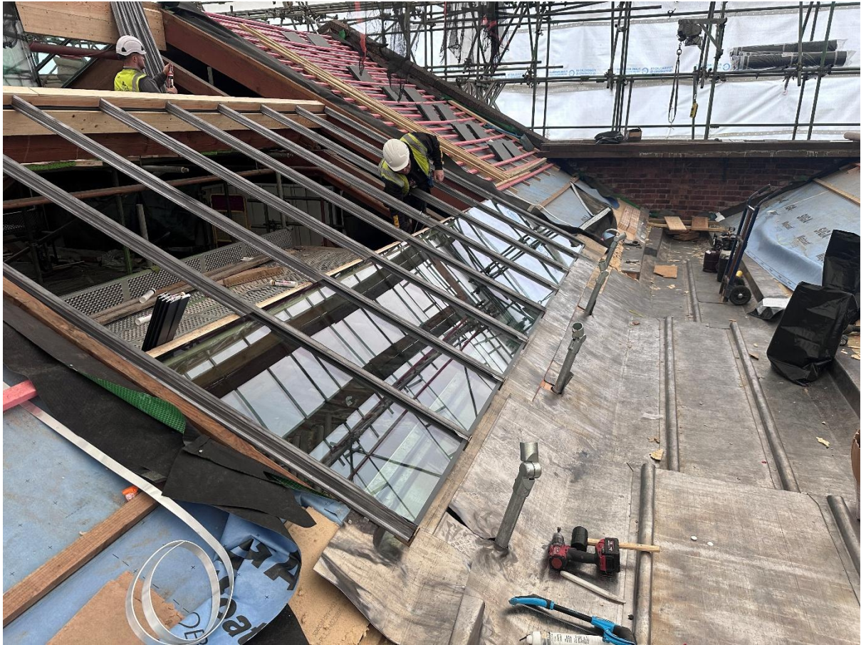
Installed fixing posts for mounting of fixed balustrading across skylight locations
