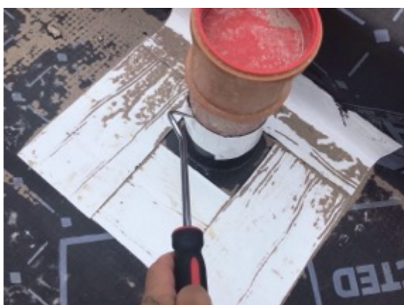
Plot 7 testing pipe seals
