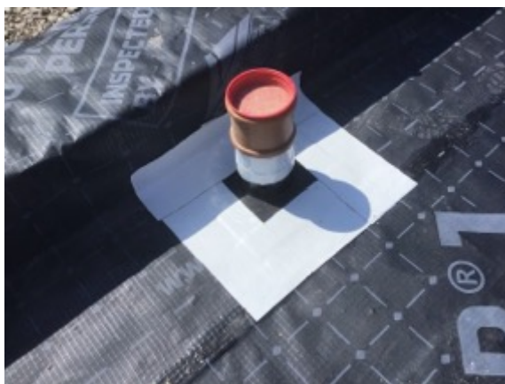
Plot 4 pipe penetration sealed with a preformed top hat and Juta GP SAM detailing
