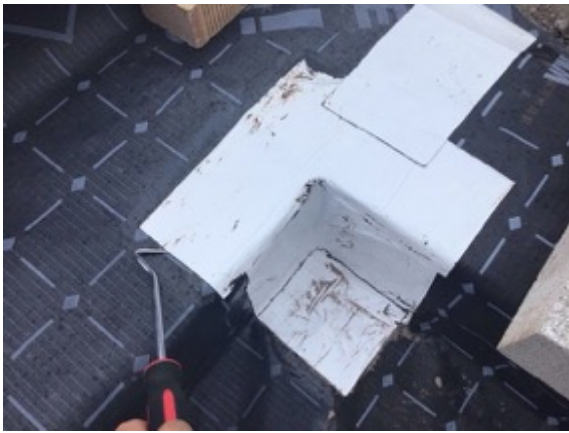
Plot 11 testing corner detailing
