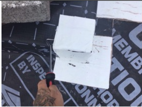
Plot 9 testing corner detailing
