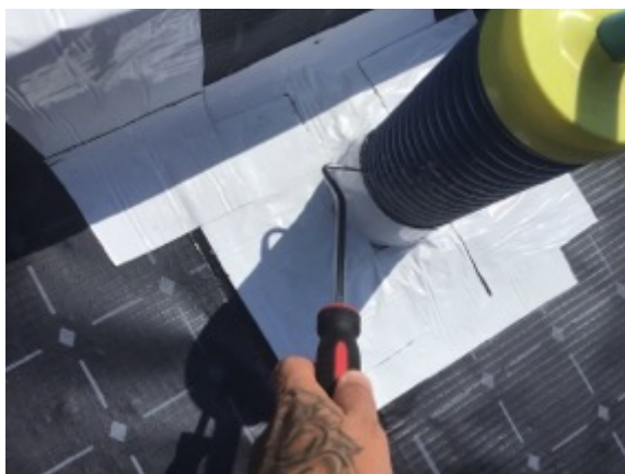
Plot 4 probe testing pipe penetration
