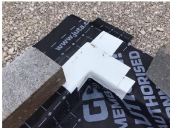
Plot 2 corner detailing sealed using Juta GP SAM and heat applied
