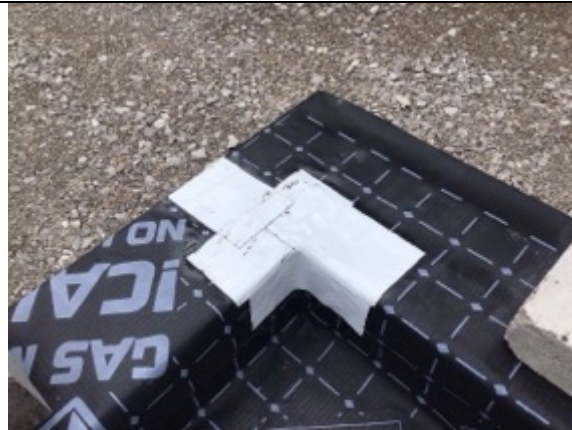
Plot 1 corner detailing sealed using Juta GP SAM and heat applied
