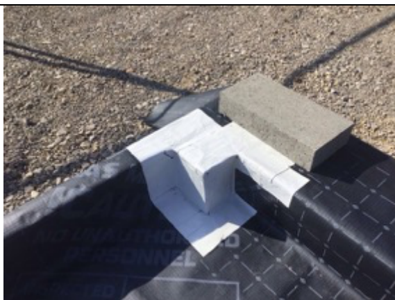
Sealed corner and threshold detailing
