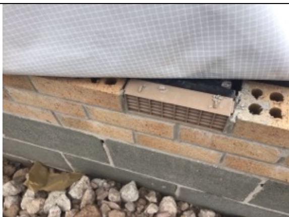
Perimeter cavity vents installed under the membrane
