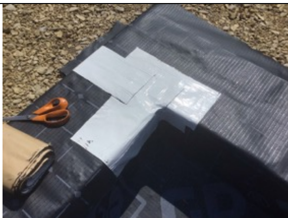
Plot 5 sealed corner detailing
