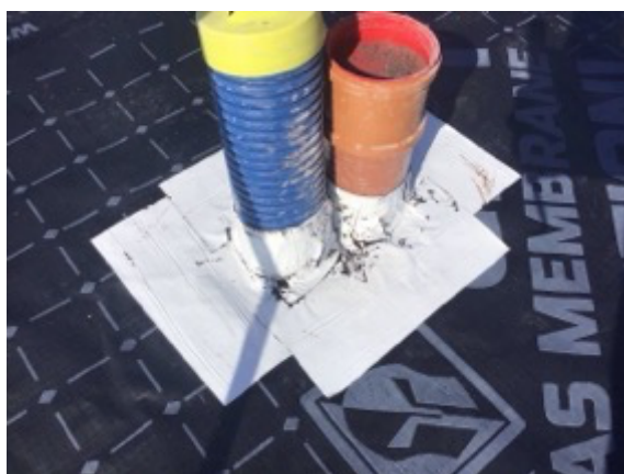
Sealed pipe penetrations
