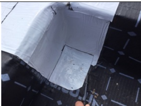
Pick testing to the sealed corner detail.
