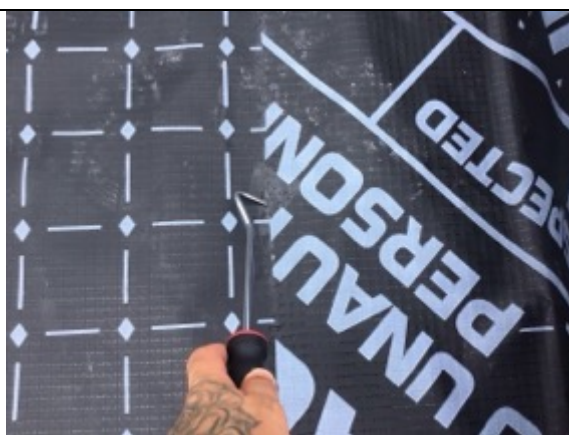
Pick testing sealed hand welded membrane lap joint
