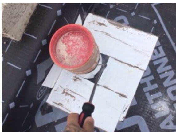
Plot 8 testing pipe seals
