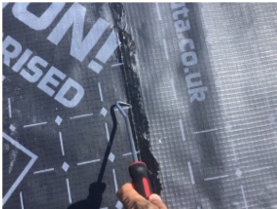
Plot 5 probe testing hand welded membrane lap joint
