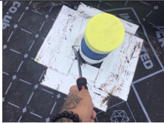
Plot 11 testing pipe seals
