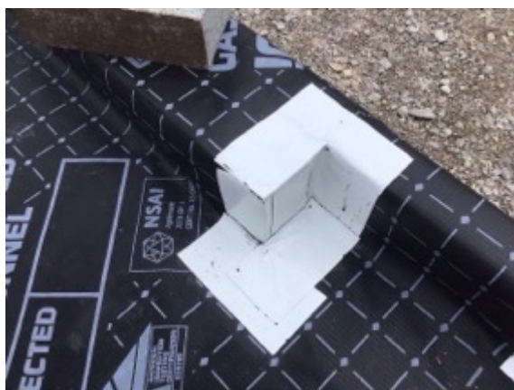
Plot 1 threshold detail sealed using Juta GP SAM and heat applied
