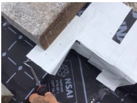
Pick testing detailing work
