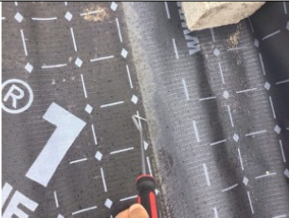
Plot 11 testing hand welded membrane lap joint
