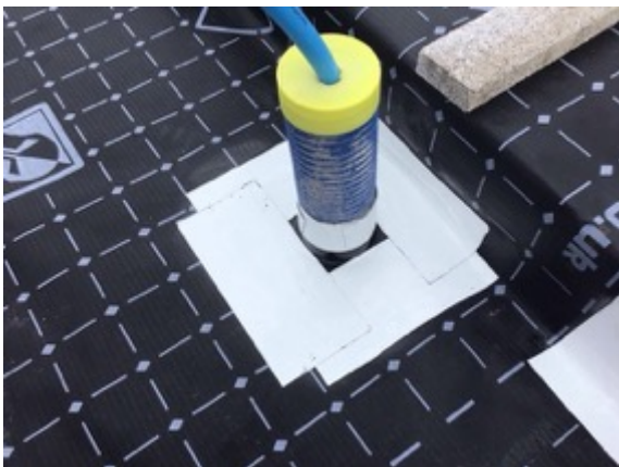
Plot 3 pipe penetrations sealed using Juta GP SAM and heat applied over a pre formed top hat
