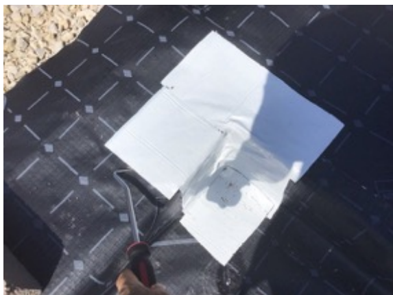
Plot 6 probe testing corner detailing
