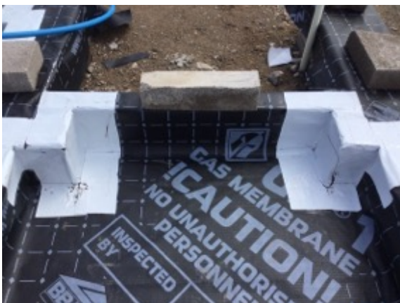
Completed threshold detail within Block 1.
