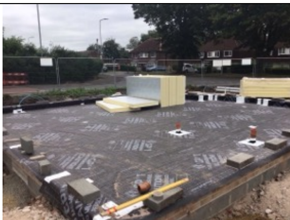
Plot 7 full line out installation
