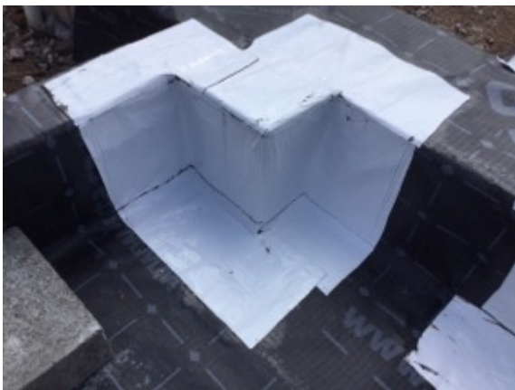
Internal corner and threshold detail sealed to Block 1.
