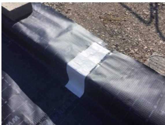
GP SAM used to strengthen the perimeter corner welding
