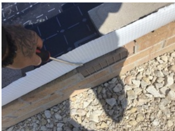
Cavity vents installed under the perimeter membrane
