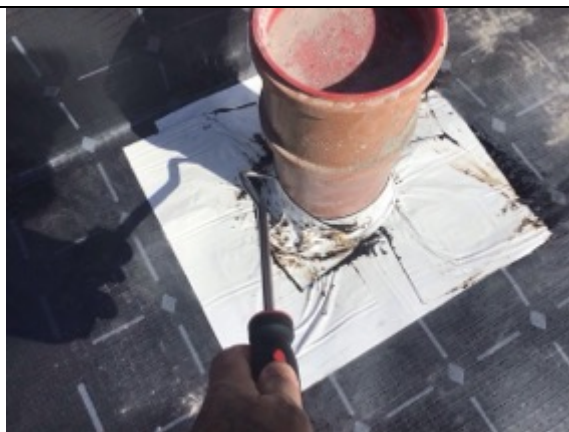
Testing sealed pipe detailing
