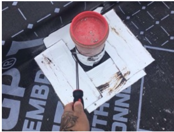
Plot 10 testing pipe seals
