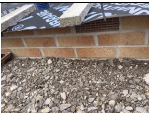
Cavity vents installed under the perimeter membrane
