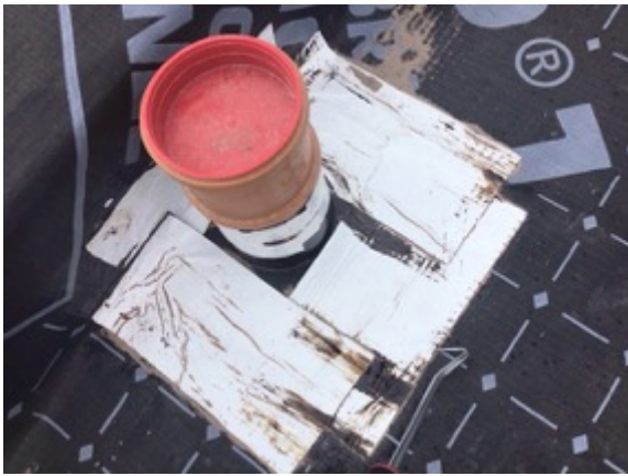
Plot 9 testing pipe seals
