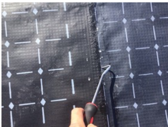
Testing hand welded membrane lap joints
