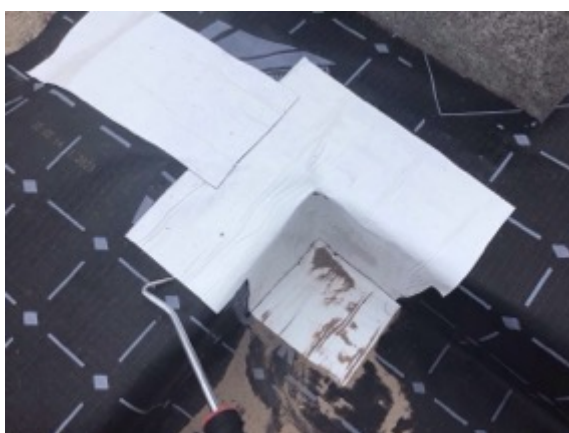
Plot 7 testing corner detailing
