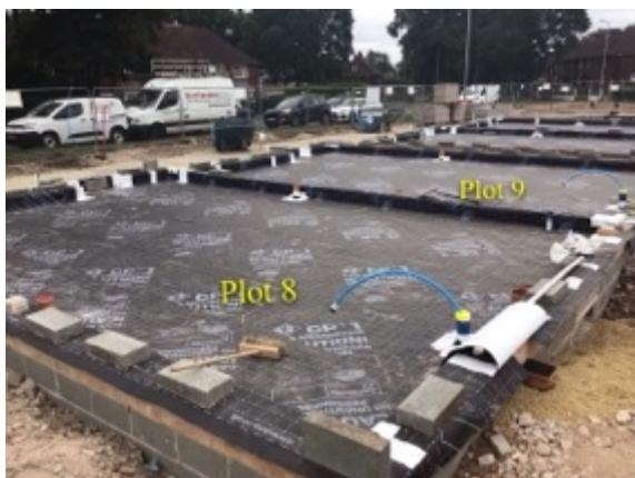
Plots 8 & 9 full line out installation
