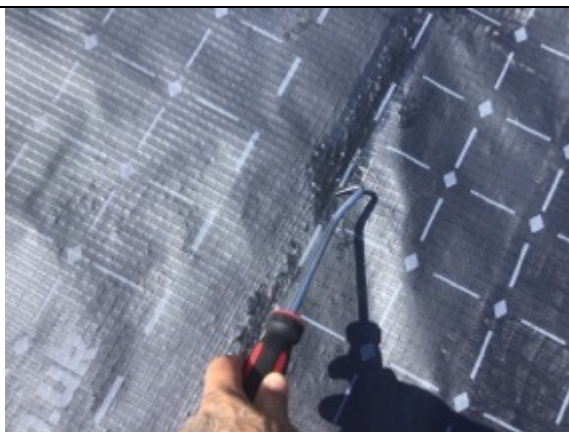
Plot 4 probe testing hand welded membrane lap joint
