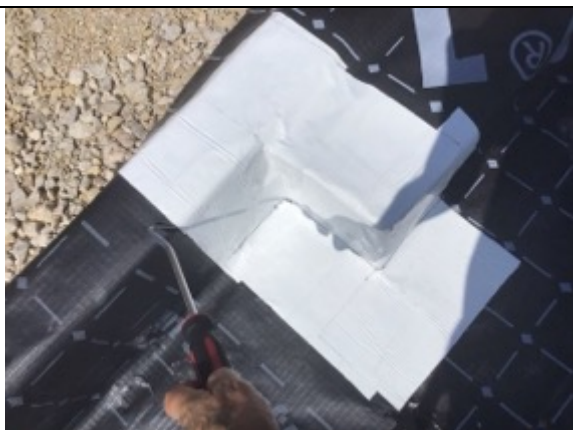
Plot 5 probe testing threshold detail
