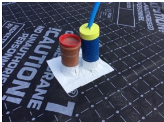
Two pipe penetration details sealed
