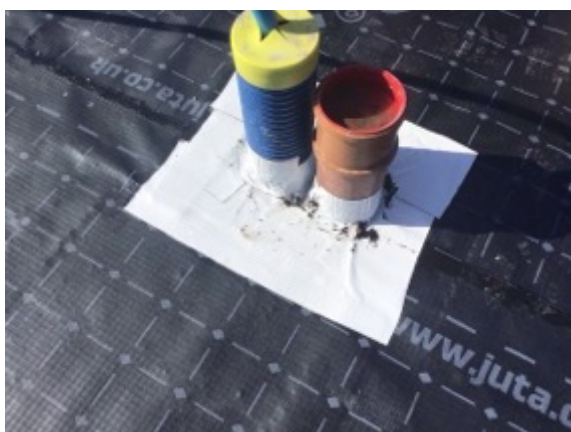
Sealed pipe penetrations
