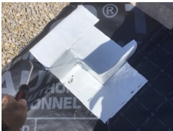
Plot 6 probe testing threshold detailing
