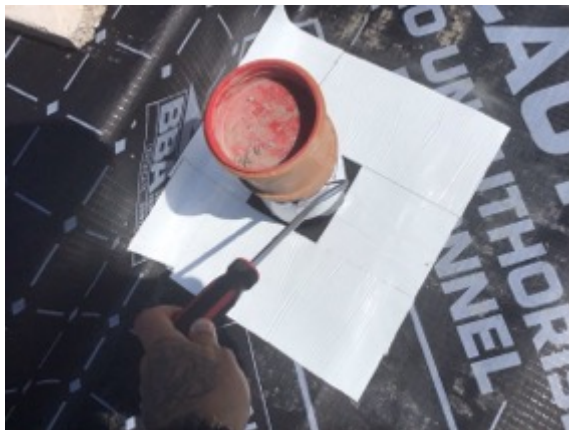
Plot 5 probe testing pipe penetration sealed with a preformed top hat and Juta GP SAM detailing
