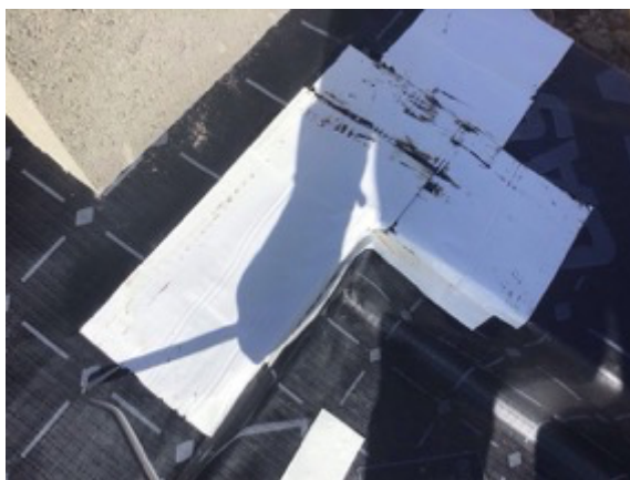
Testing corner detailing
