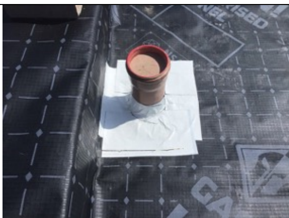
Plot 6 pipe penetration sealed using Jута GP SAM
