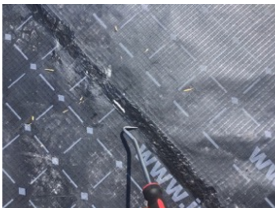
Plot 6 probe testing hand welded membrane lap joint
