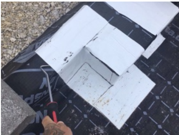
Plot 10 testing threshold detailing
