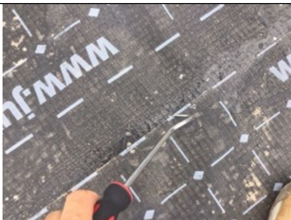
Plot 7 testing hand welded membrane lap joint
