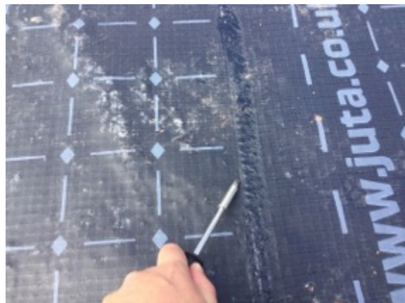
Pick testing along the welded lap joint.
