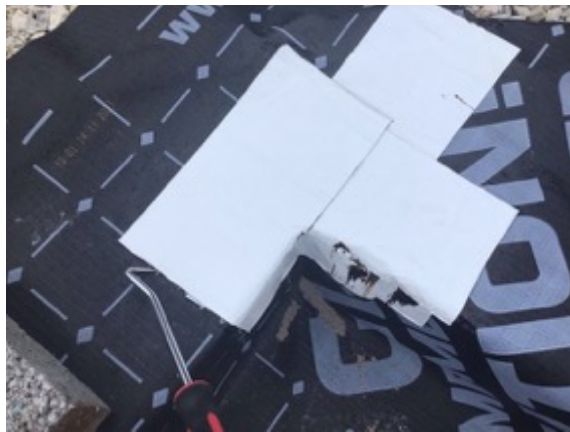
Plot 10 testing corner detailing
