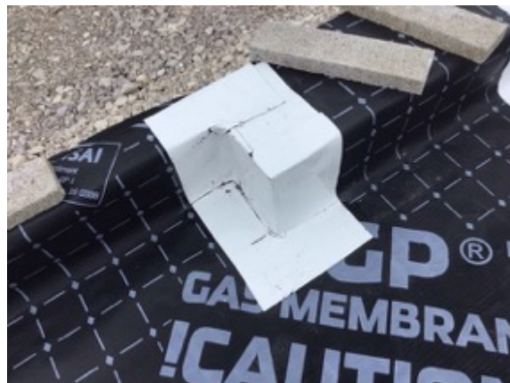
Plot 3 threshold detailing sealed using Juta GP SAM and heat applied
