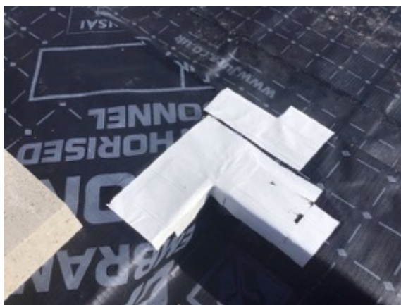
Sealed corner detailing
