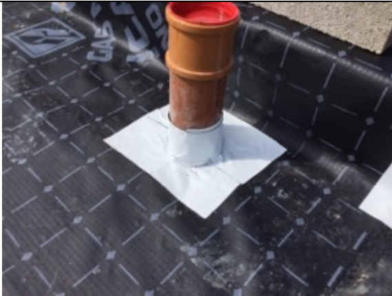
Close up of the pipe penetration detail sealed.
