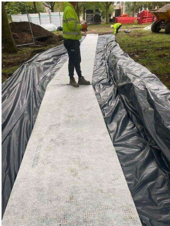
Figure 5 – Permeable Paving Installation
