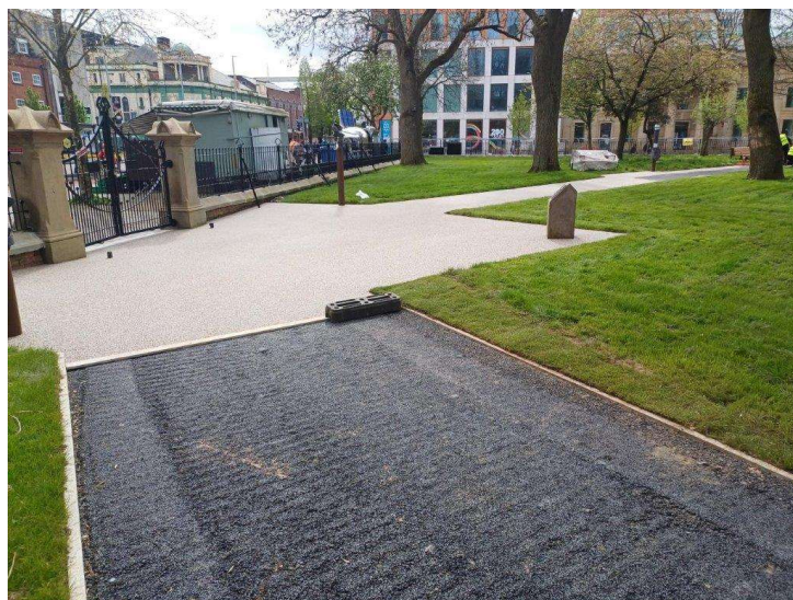
Figure 8 – Permeable Paving Installation
