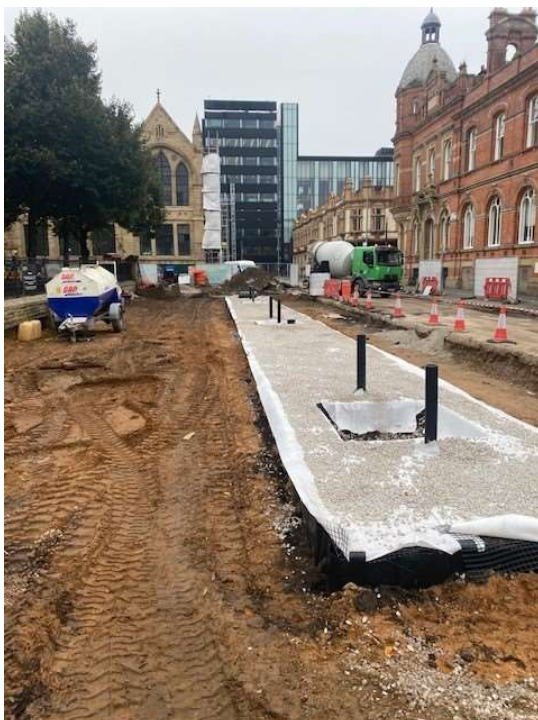
Figure 12 – Tree Pit Installation
