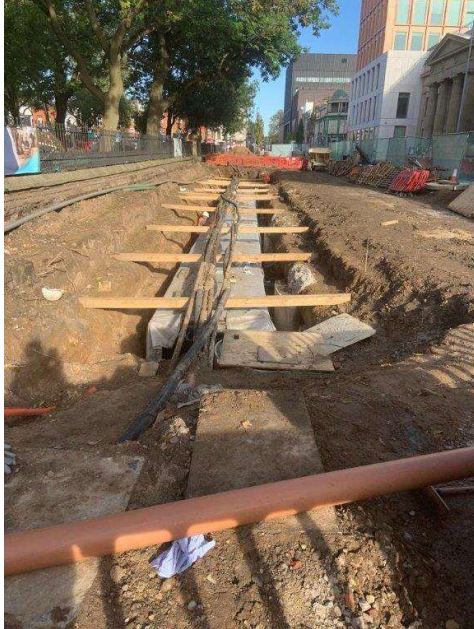
Figure 4 – Tank Installation
