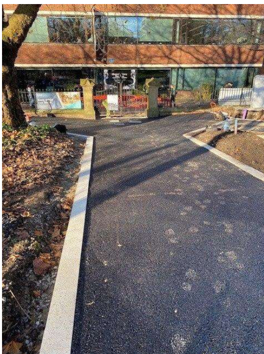
Figure 7 – Permeable Paving Installation
