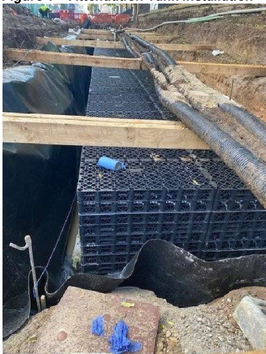
Figure 1 – Attenuation Tank Installation
