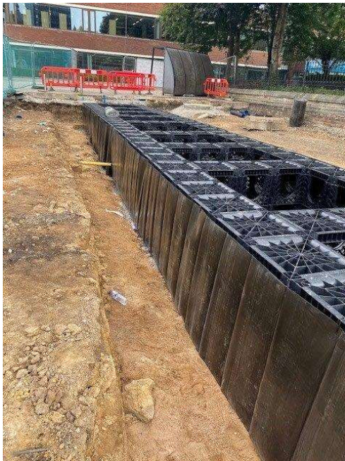
Figure 12 – Tree Pit Installation
