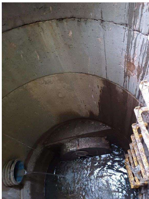
Figure 9 – Flow Control Installation
