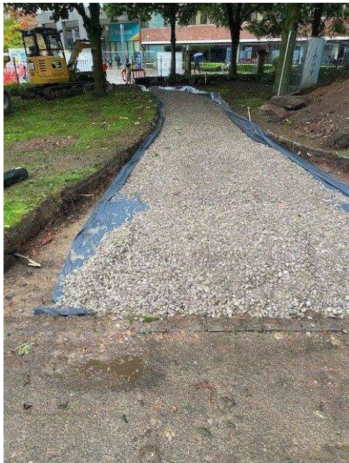
Figure 6 – Permeable Paving Installation
