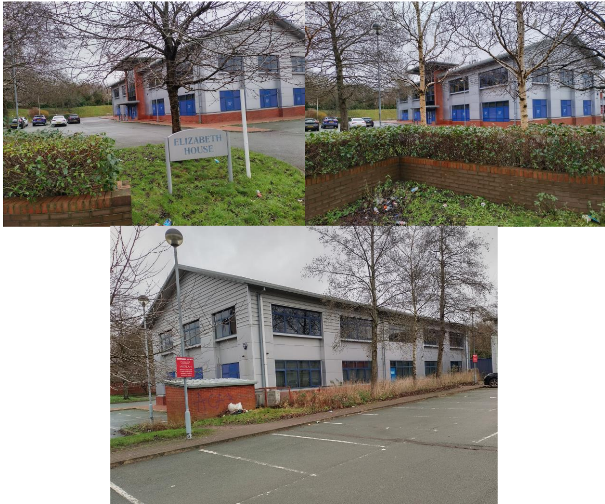
Fig.1 – Views of the application site.
