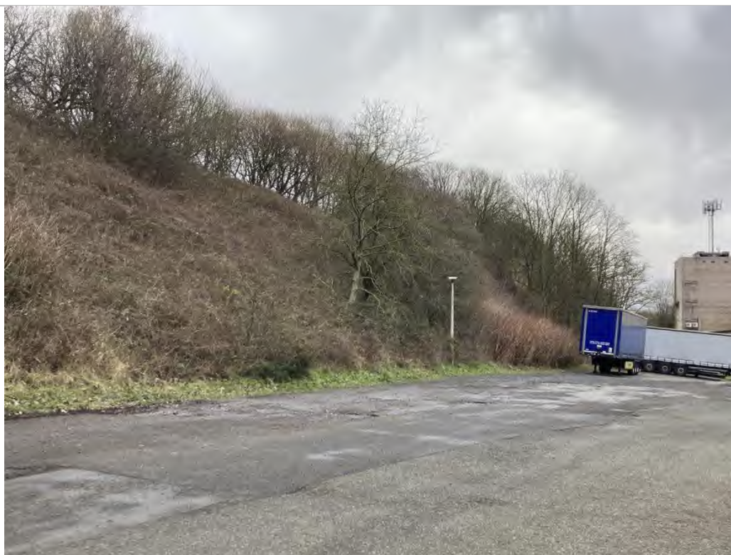
PLATE 8 RETAINING WALL AND SLOPE ALONG THE NORTHERN BOUNDARY
