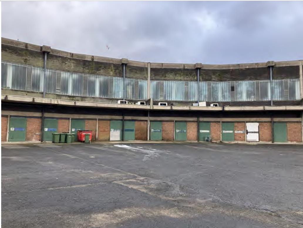
PLATE 10 INSIDE THE CENTRAL BUILDING ON SITE
