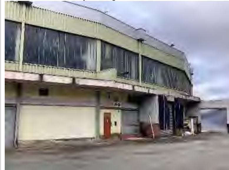
Central former butchery building:
