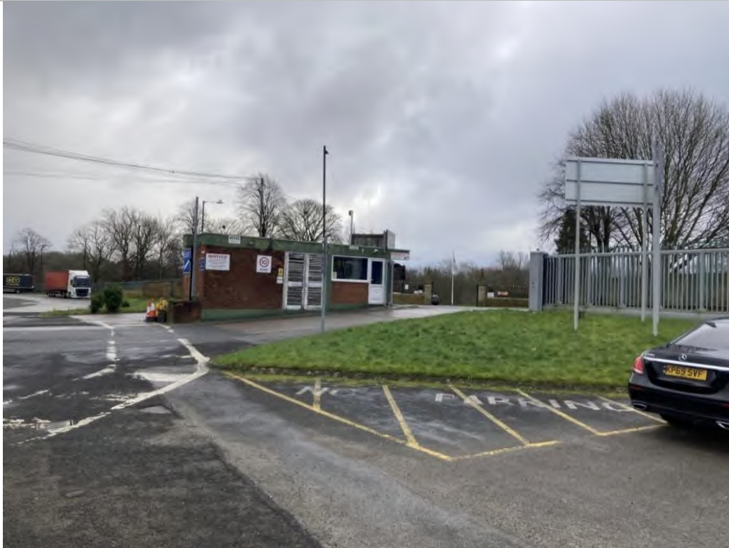
PLATE 9 ELECTRICAL SUBSTATION AT THE SITE ENTRANCE
