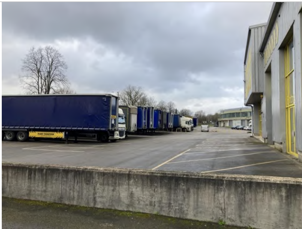
PLATE 2 SMALL RETAINING WALL IN THE EAST OF THE SITE
