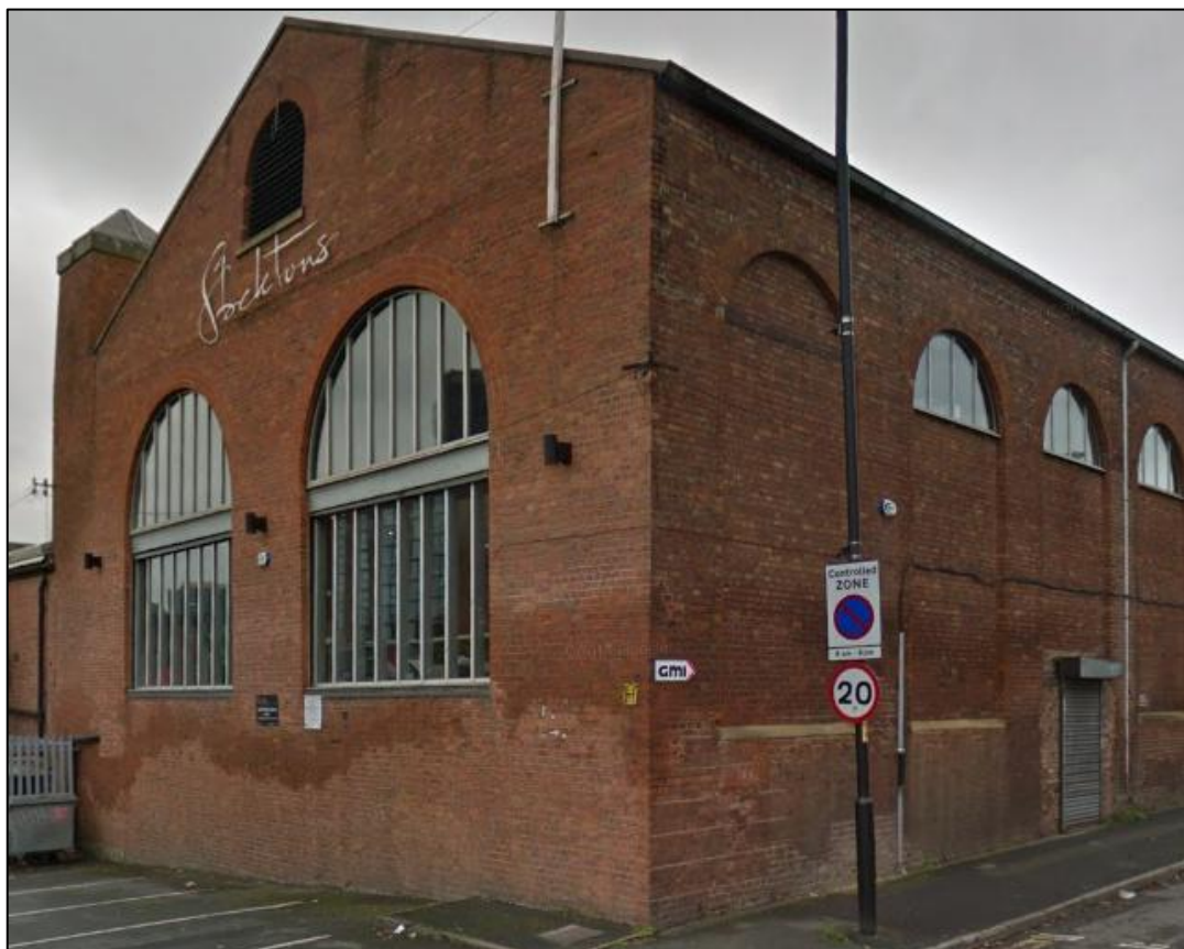
Plate 20 View of 19th-century works at Ducie Street (formerly Mather Street), with view matching that seen in the 1902 photograph of Mather Street
