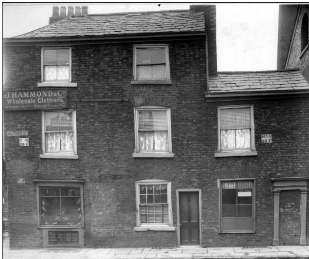
Plate 12 No. 40 Mather Street and No. 136 Gt. Ancoats Street, with chimney of the Iron & Steel Warehouse visible in the background, 1902
