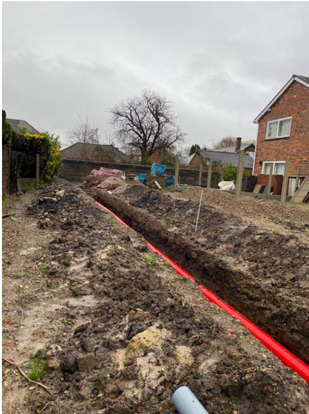
Image of cable
