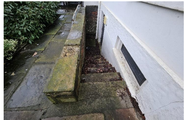
Figure 13: Basement Steps to front entrance
