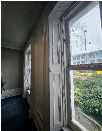
Figure 18: View onto Oxford Rd.
