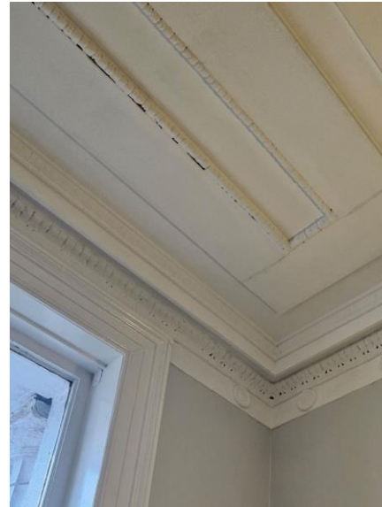
Figure 16: Cornicing to Room G.007a
