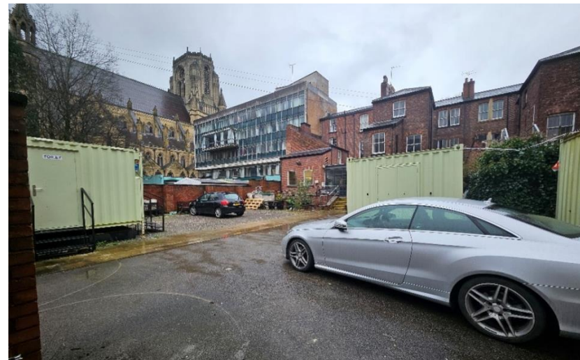
Rear of the building
