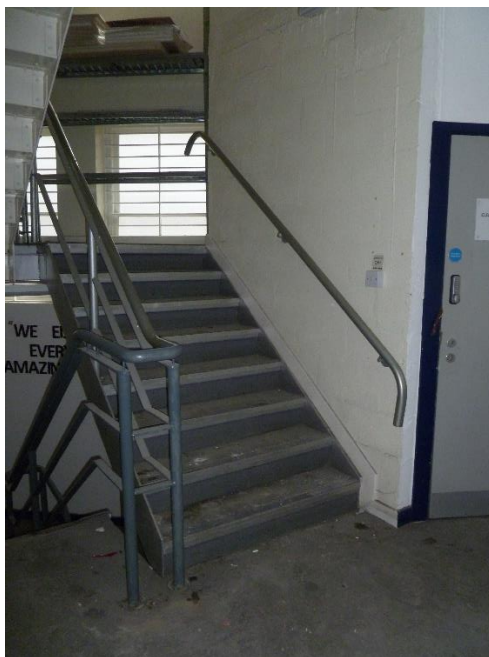
Inserted staircase leading to all floors.
