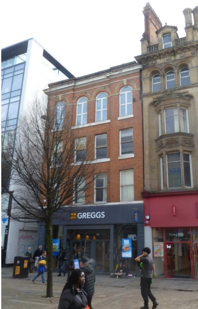
Figure 2.1: View of the building from Market Street.
