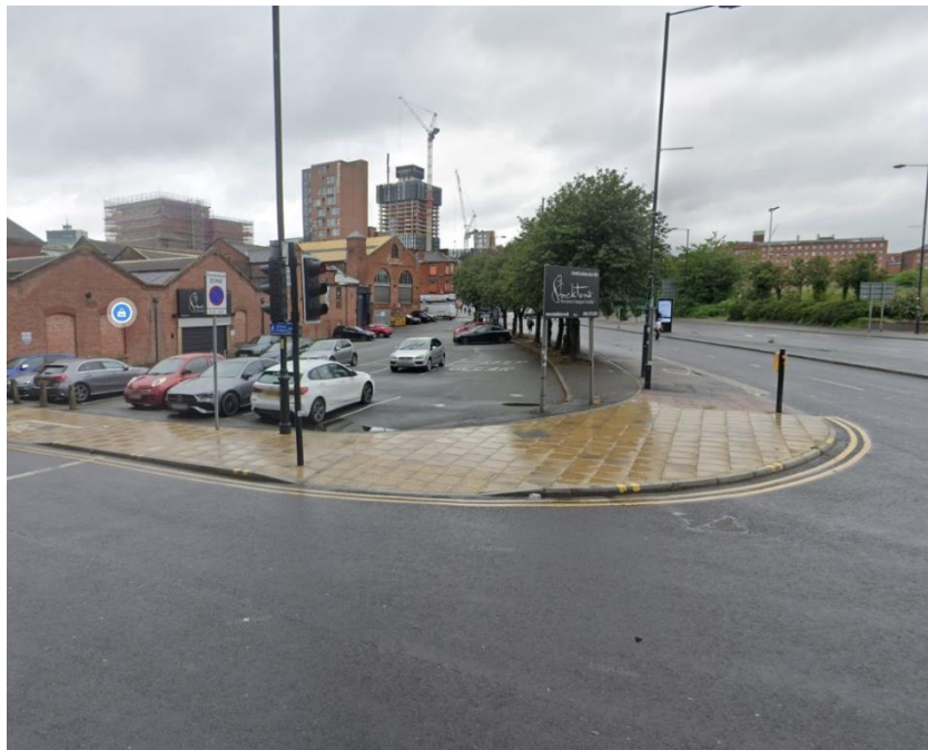
Figure 2.3: The site at the junction of Store Street and Great Ancoats Street looking north
