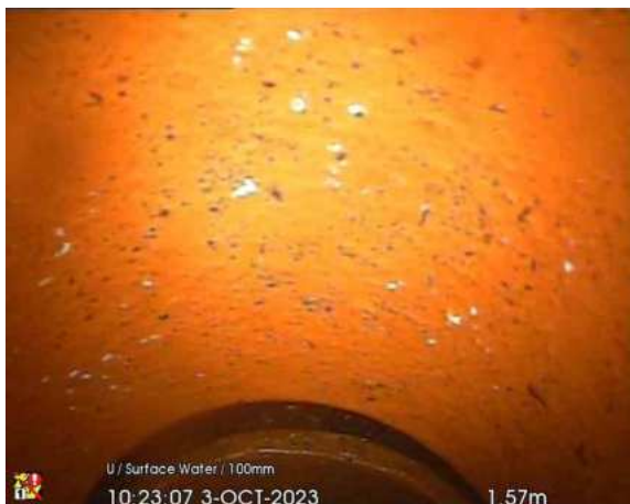
MH28 US RWP A_1-57m_102307.jpg, 00:00:32, 1.57 m Open joint, medium
