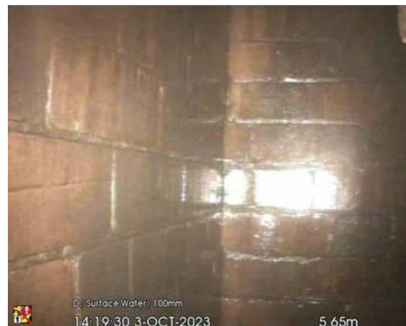
MH4A DS MH5_5-65m_141930.jpg, 00:00:33, 5.65 m Finish node, manhole, reference: MH5, CULVERT MH
