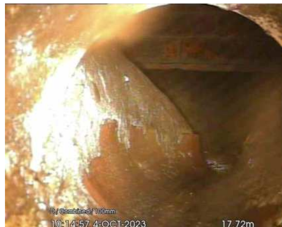
MH24 DS_17-72m_101457.jpg, 00:01:15, 17.72 m Finish node, manhole, reference: DS, UNCHARTED, POSS UNDER CABINS
