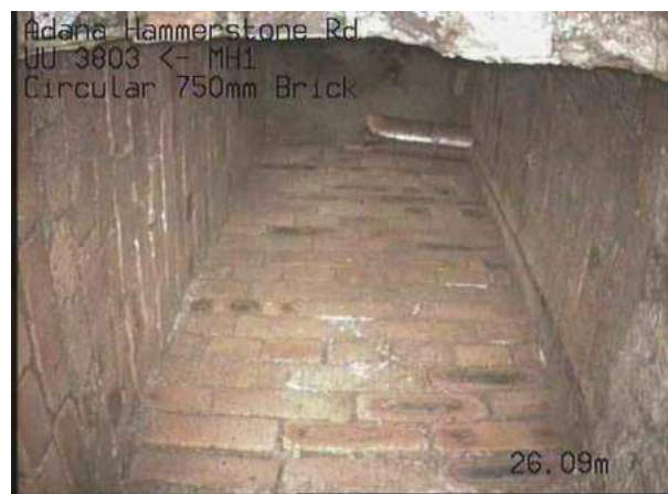
UU 3803X_7c8327ac-b3ef-4fae-86ac-5e048638f9f8_20230929_110857_666.jpg, 00:03:18, 26.09 m Start node, manhole, reference: Node point, 150mm pipe incoming
