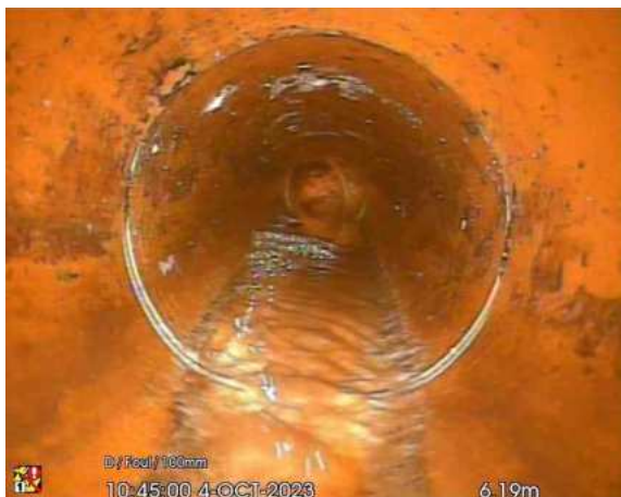
FWIC1 DS MH25_6-19m_104500.jpg, 00:00:27, 6.19 m Water level, 20% of the vertical dimension, DIP
