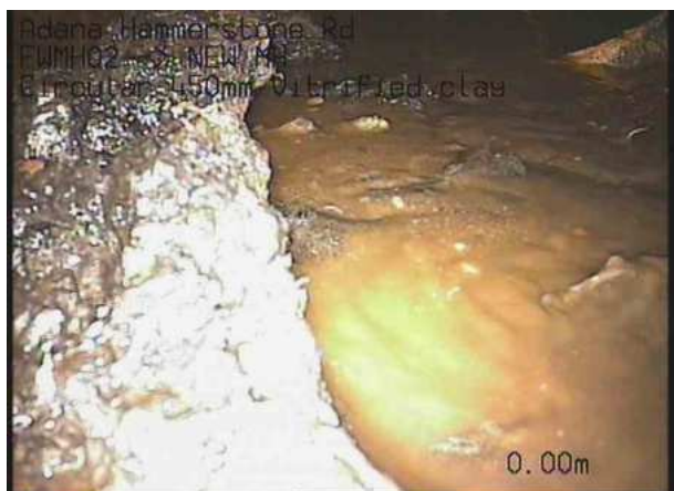
FWMH02X_db9322b8-9ab3-4d4a-8258-9b1e2f5a8361_20230929_124453_432.jpg, 00:00:00, 0.00 m Start node, manhole, reference: FWMH02, Hard standing in MH
