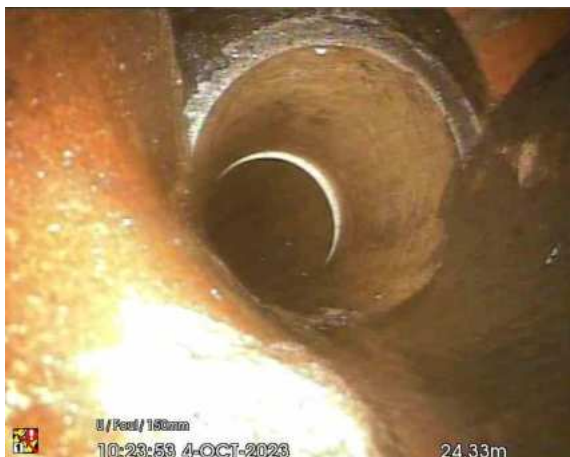
MH25 US_24-33m_102353.jpg, 00:01:47, 24.33 m Finish node, manhole, reference: US UTL
