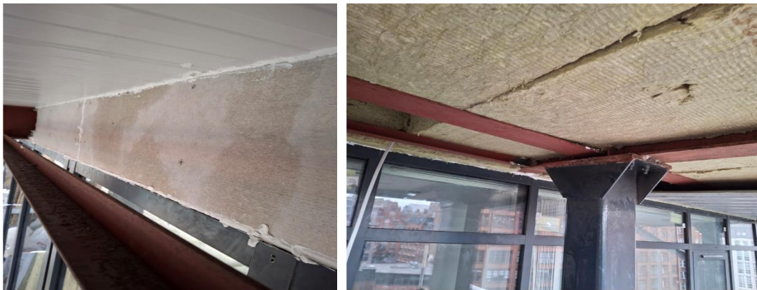
Photographs showing Remedial Works undertaken to Profiled Roof
