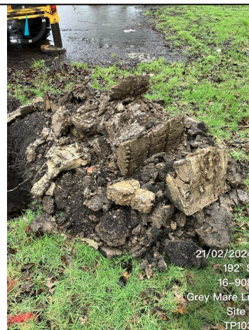
Trial Pit 103 Spoil
