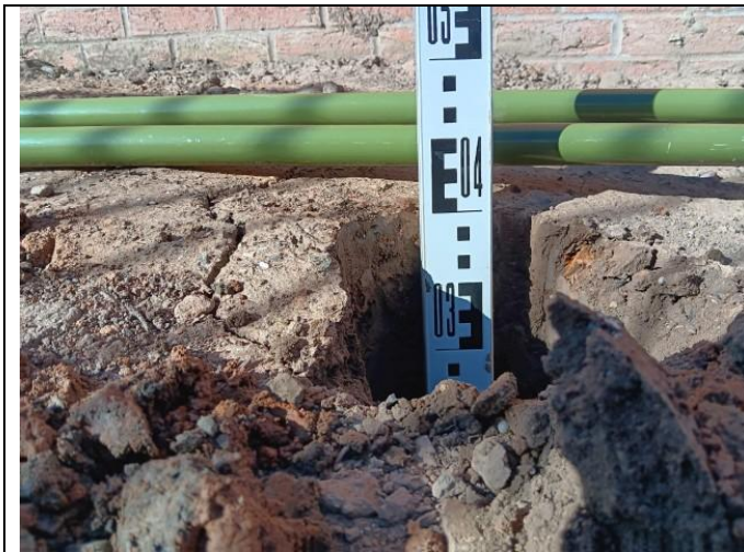
Photograph 7: Evidence of suitably chemically validated topsoil with a minimum of 150mm growing medium in the soft landscaping area surrounding the apartment block (area 3) over pea gravel.
