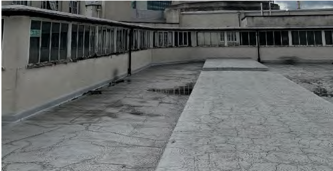
Figure 18: Bitumen - Seventh Floor
