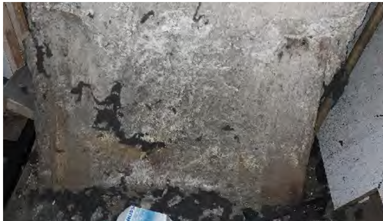
Figure 1: Gusset Plate - Basement
