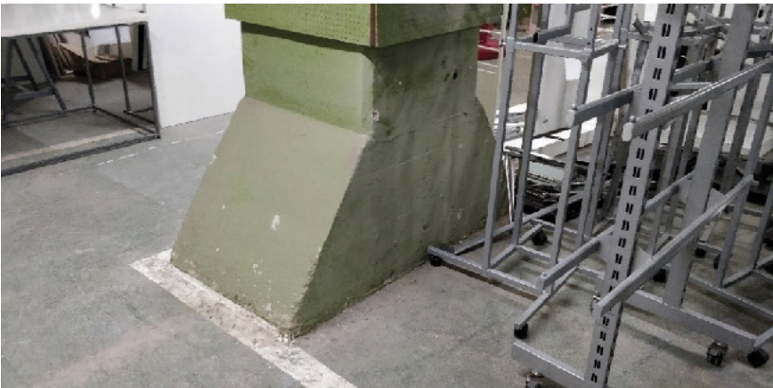
Figure 2.5: Splayed Columns
