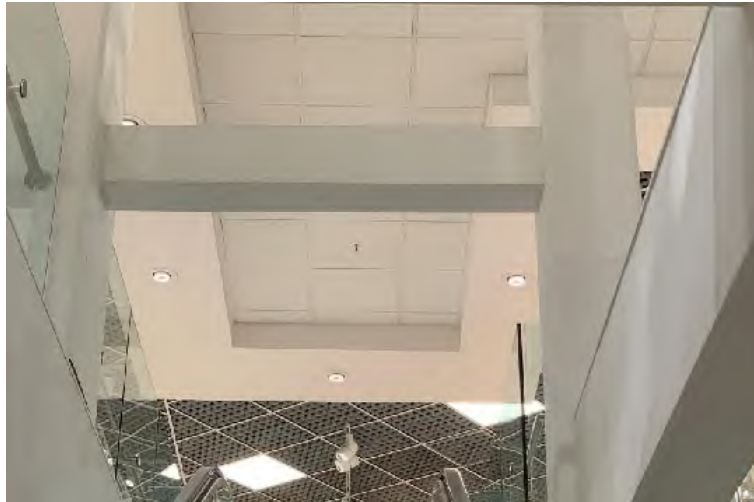
Figure 2: Escalators - Third Floor
