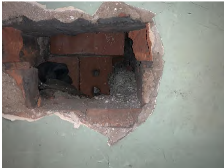
Figure 7: Opening Up Works - Fifth Floor
