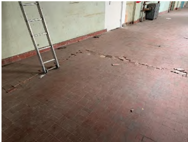
Figure 15: Tiled Floor - Seventh
