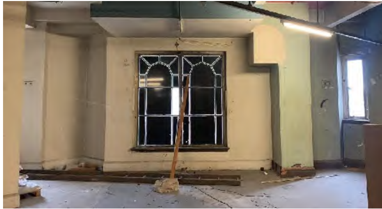
Figure 8: Windows - Fifth Floor
