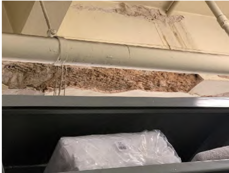
Figure 4: Beam Encasement - Fourth Floor
