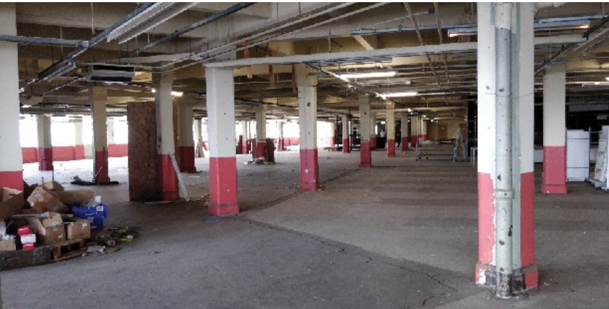
Figure 2.4: Splayed Columns
