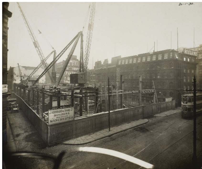
Figure 2.2: Historic Photograph of Rylands Building Under Construction
