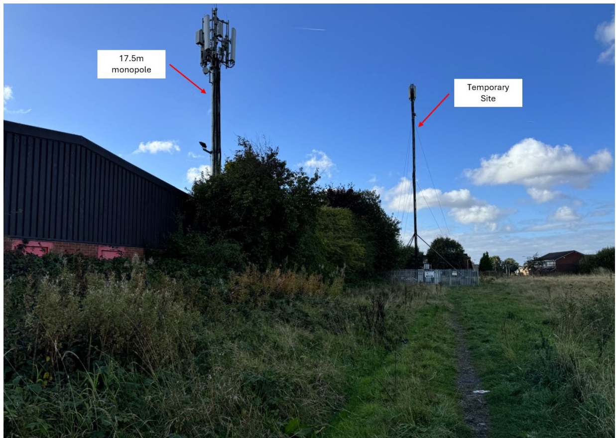
(Figure 1: The existing 17.5m pole which is being replaced and the temporary site which will also be replaced. Source: Taken from site visit)
