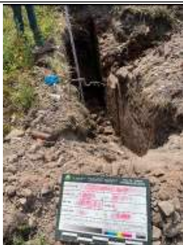
Pit C: View of excavation
