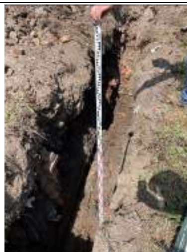
Pit A: View of excavation
