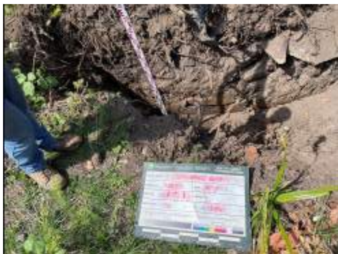
Pit B: View of excavation
