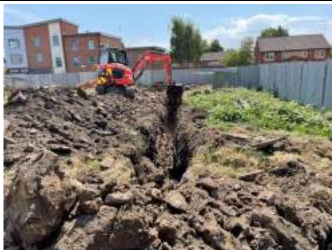
Trench 5A: View of excavation
