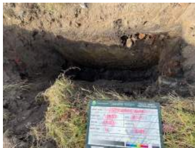
Soak Away 1: View of excavation
