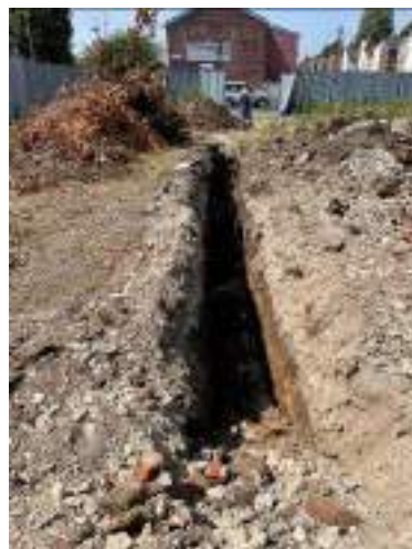
Trench 3: View of excavation
