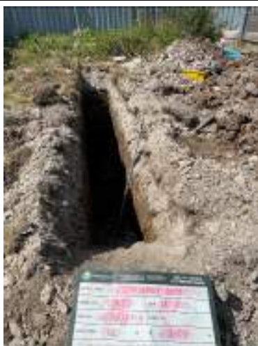
Trench 4: View of excavation
