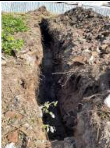
Trench 5B: View of excavation
