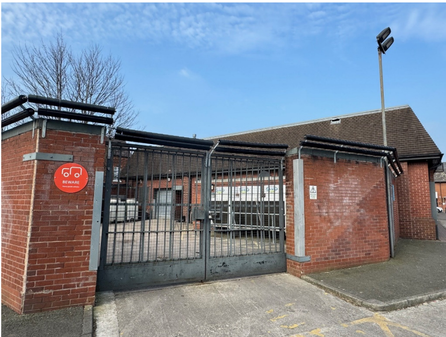
Plate 8 – Secure entry gates from car park to service yard . These will remain unchanged and will be a communal entry point for both units .
