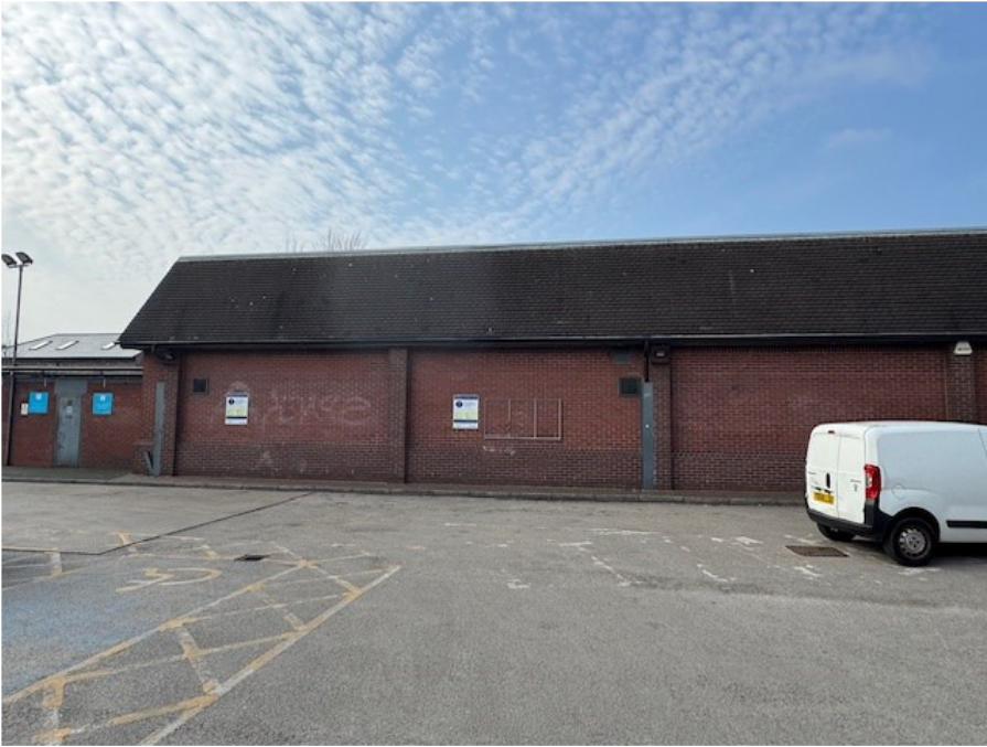
Plate 3 – Side elevation facing the car park. New shop front to these three brick bays providing primary access to unit B
