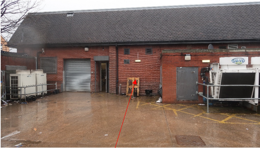
Plate 9 – Rear Elevation and Service Yard . This will become a communal area for the two units . All plant and equipment will be removed . A fire exit door for unit B will be provided (arrowed red)
