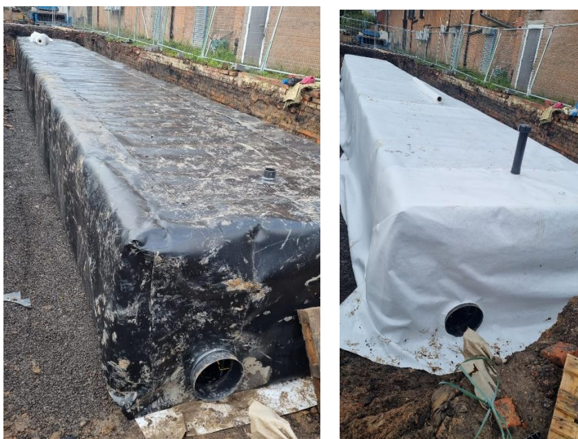
Fig 5 - Cell construction underway – Tanks 1&2
