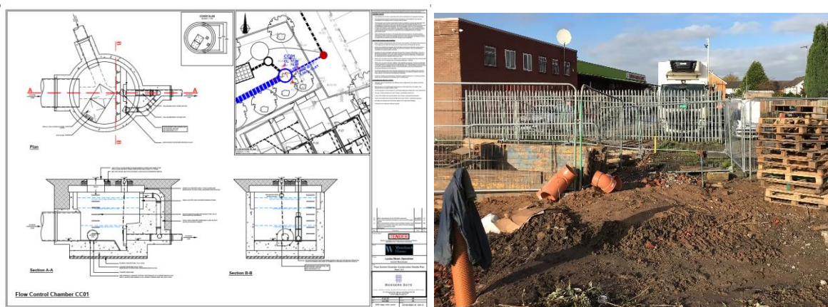
Fig 3 Design and construction underway of Manhole CC01, hydrobrake control chamber.
