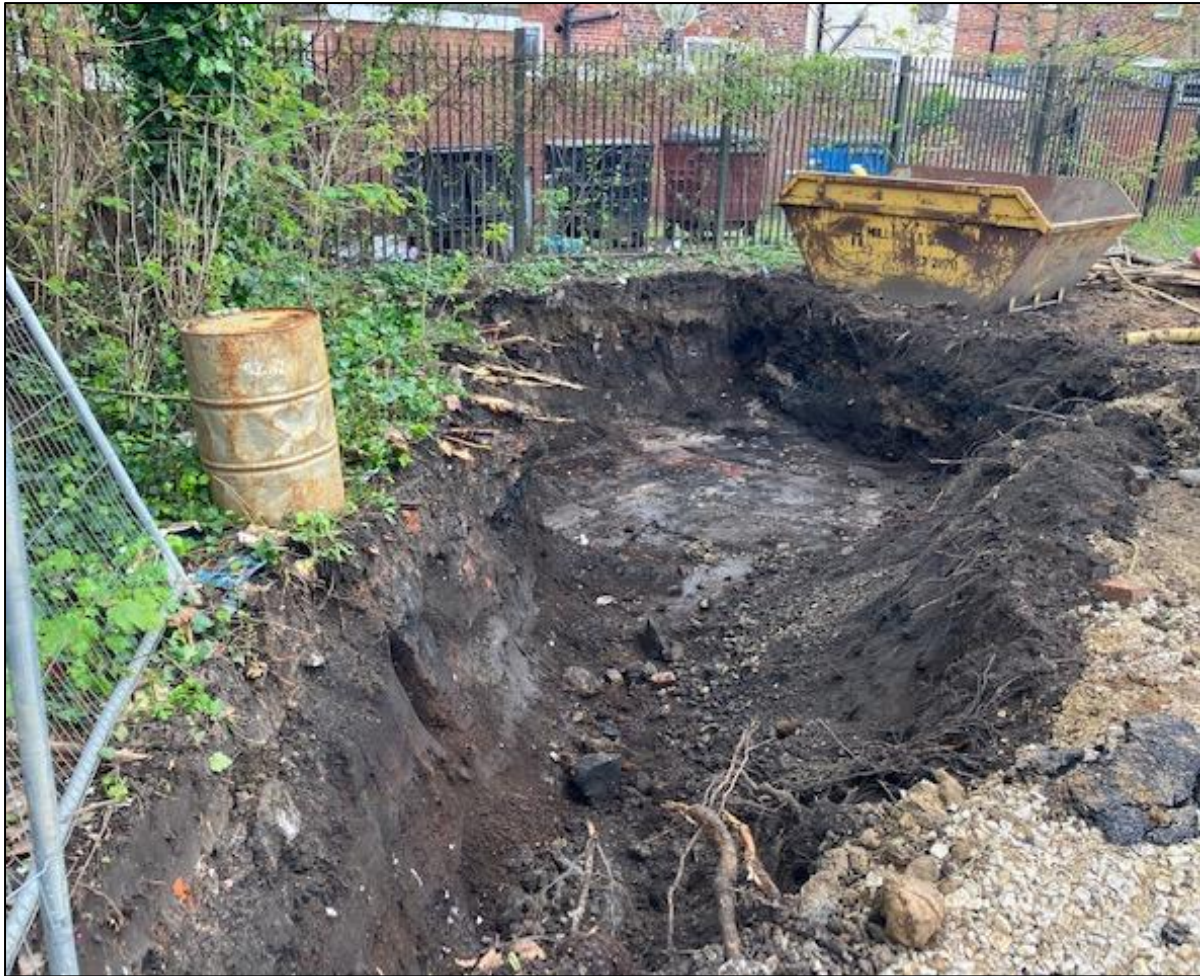
Figure 1 – The area of the excavation around TT01.
