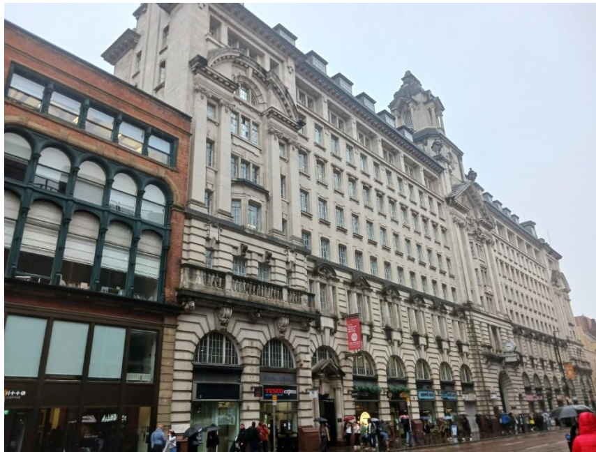
Figure 2.2: View of St James Building from Oxford Street.
