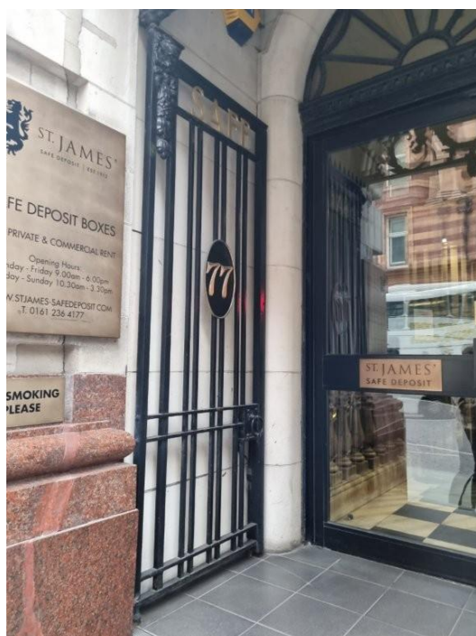
Image 5.1 Left hand gate and existing door
