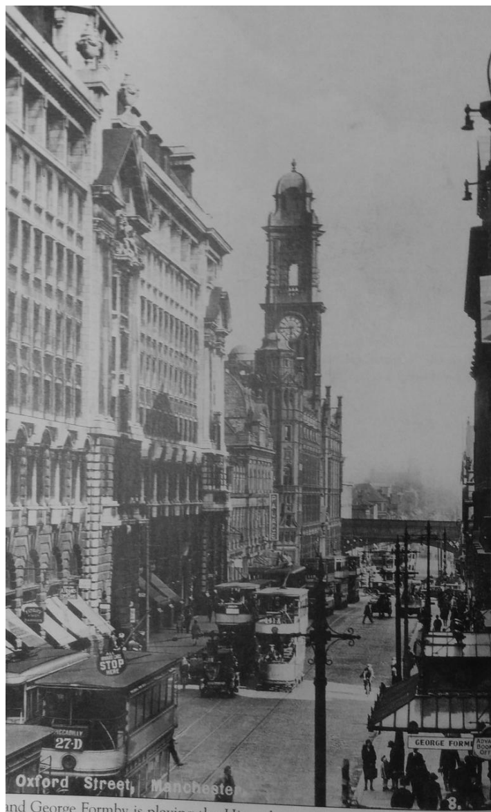
Figure 2.5: St James's Buildings c.1932 with the Palace Theatre in the background (Stewart 2004)
