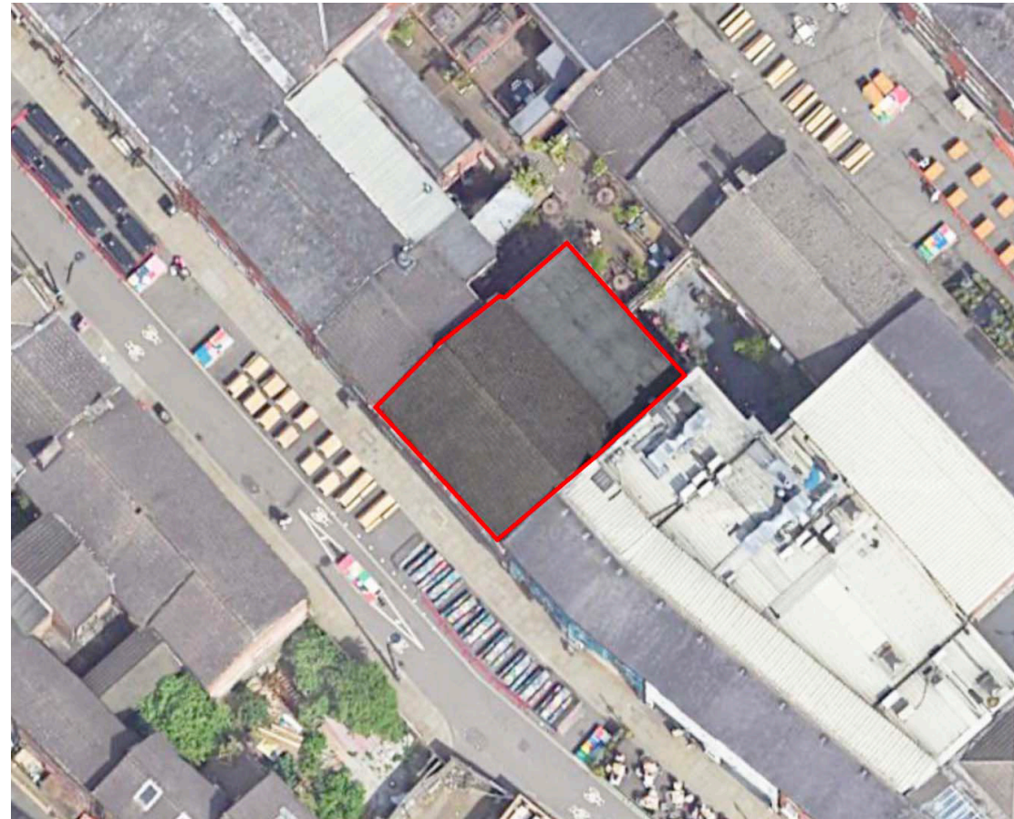
Aerial view with the application building outlined in red
