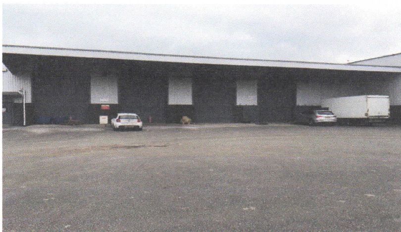
Photograph 1.7 Main drainage in middle of the yard.
