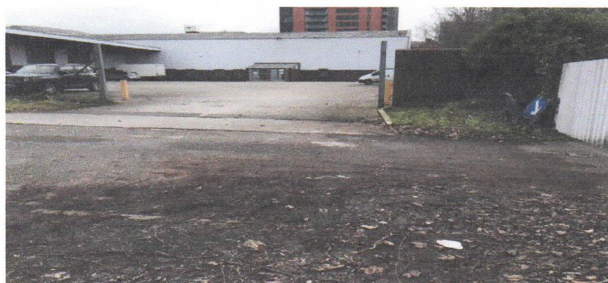
Photograph 1.5 The entrance to site from Mary Street, which is rising away from the river to the right of picture.
