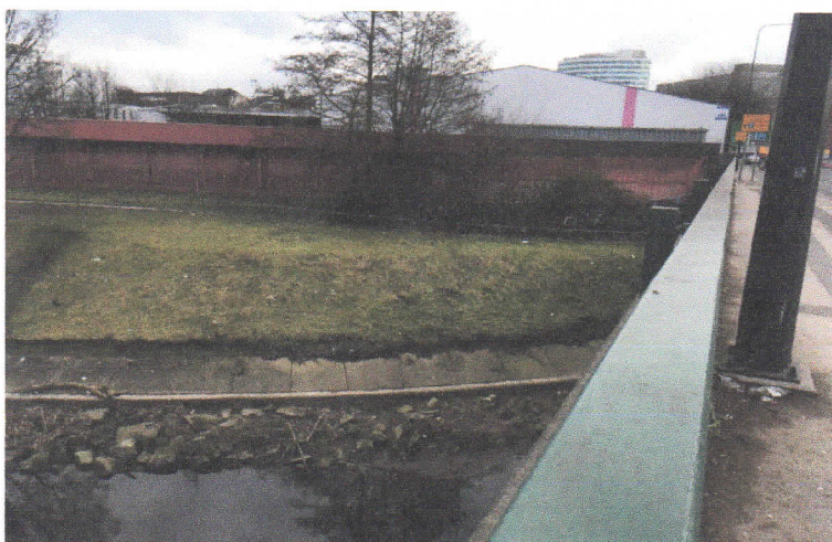
Photograph 1.3 Site building in the foreground with Trinity Road and bridge to the right. River and river bank to the foreground.
