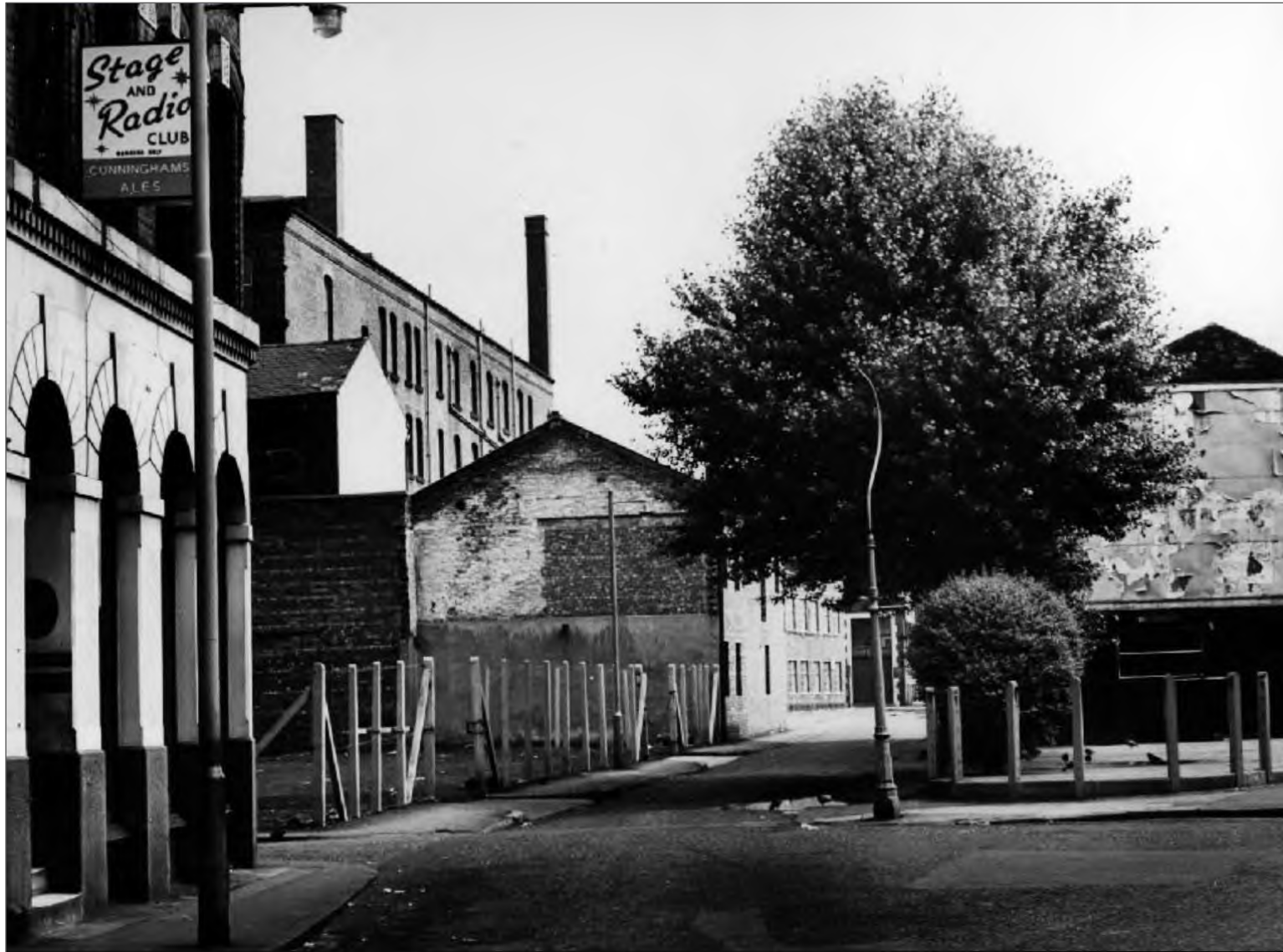
Plate 2: Photograph of the Site taken from the junction of Dean Street and Port Street in 1966 [Manchester Libraries, m01431]
