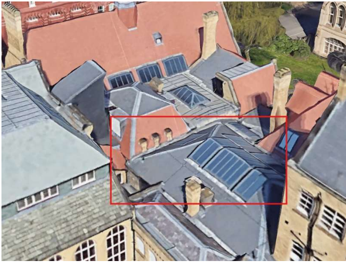
Location of new ladder and walkway – not visible from ground level*
