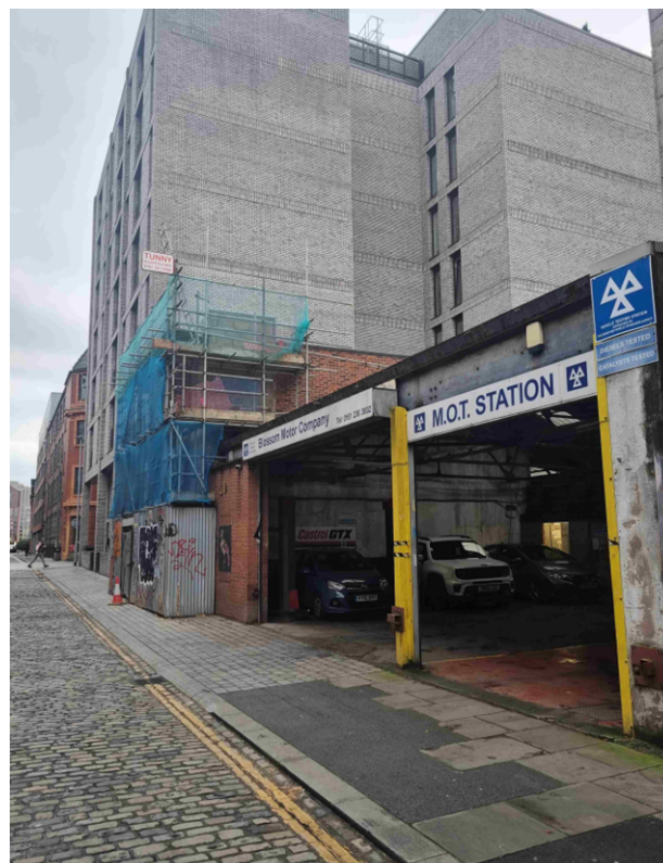
The site with neighbouring two storey commercial unit currently under construction, and 8no storey apartment building at no13 Blossom Street in the foreground, pictured from Henry Street facing south-east
