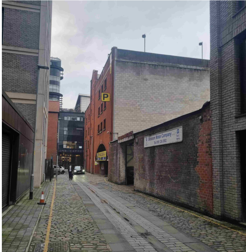
The site, with neighbouring four storey car park and Grade II listed Express Building in the foreground, pictured from Gun Street facing north-west.
