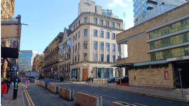
View eastwards of the building from Peter Street
