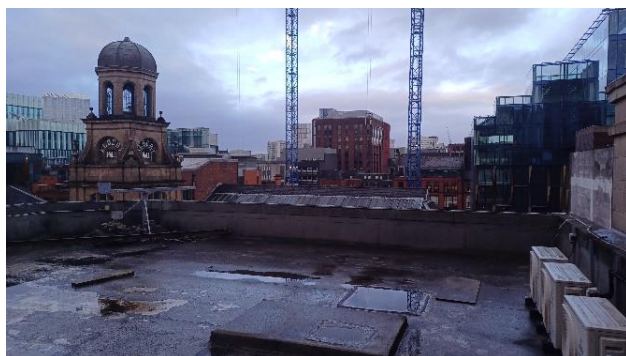
View northwards from the roof terrace showing AC units and parapet
