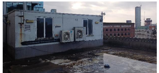
View of the plant room from the roof terrace
