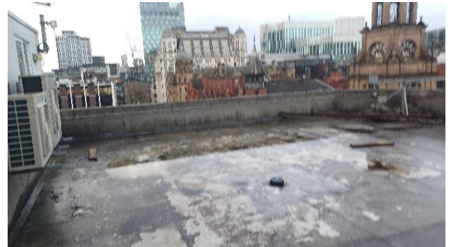
View westwards from the roof terrace with plant room and wall mounted AC units on the left
