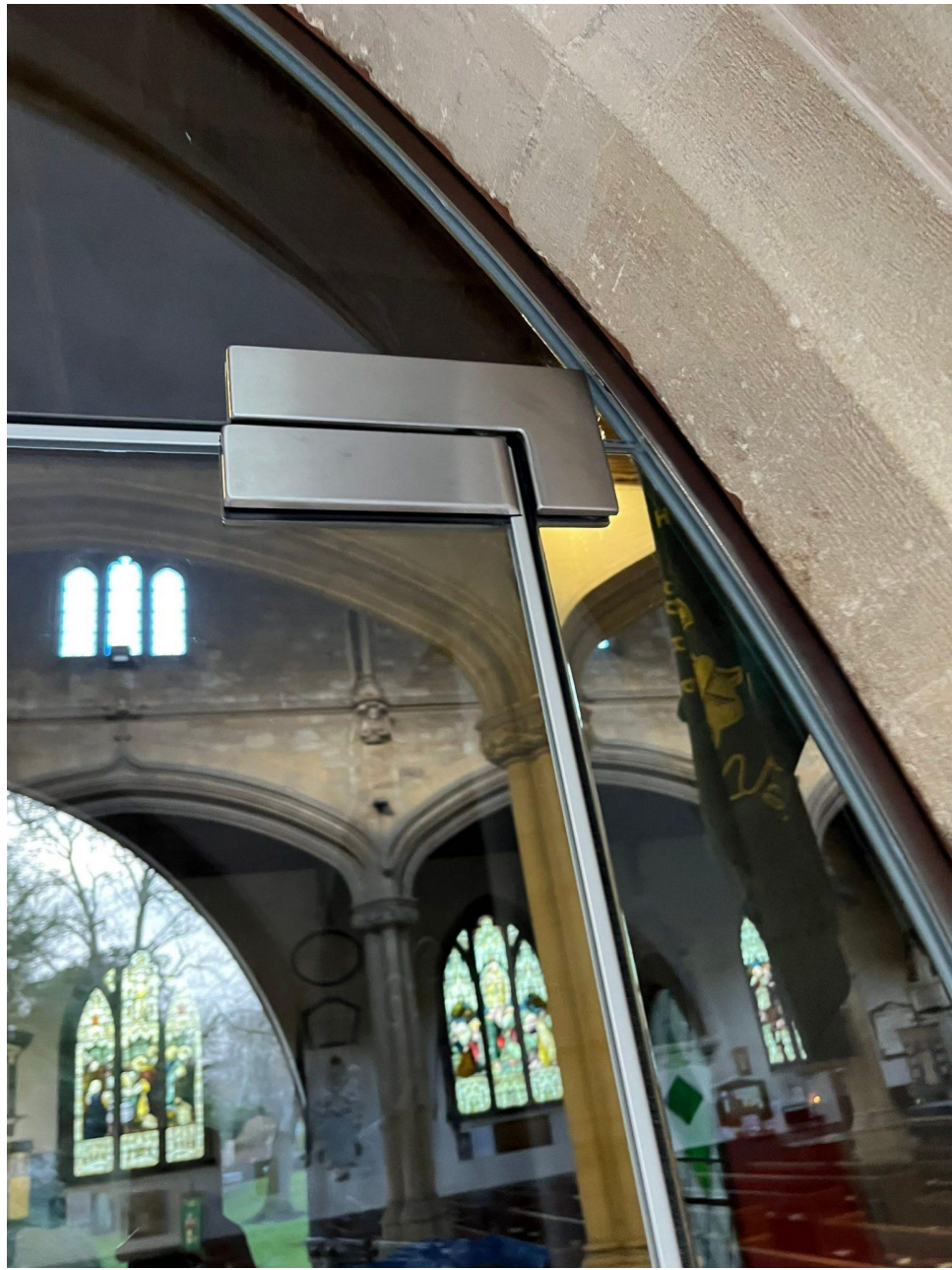
A PROPOSED FRAMELESS GLAZING PERIMETER DETAIL
