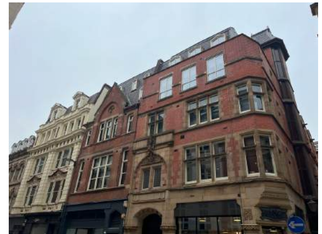
2.8 View of Site roofing from South King Street.heic
