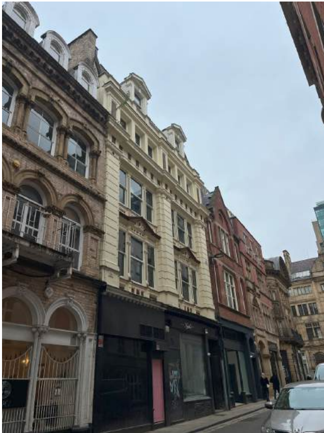
2.9 Roofing from South King Street.heic
