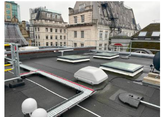
2.16 View of modern skylights and services on roof.heic
