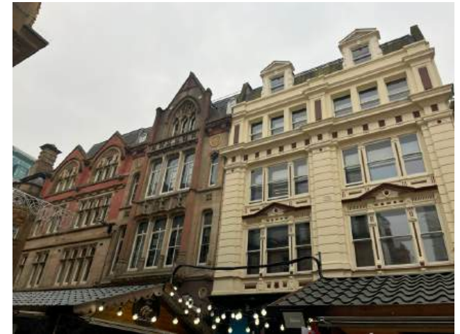
2.7 View of site roofing from King Street.heic
