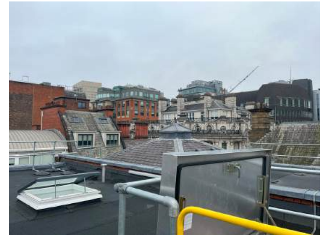
2.15 View East across roofscape from hatch entrance.heic
