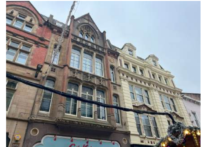
2.11 Mansard roof visible from street level directly viewing roof space on King Street.heic
