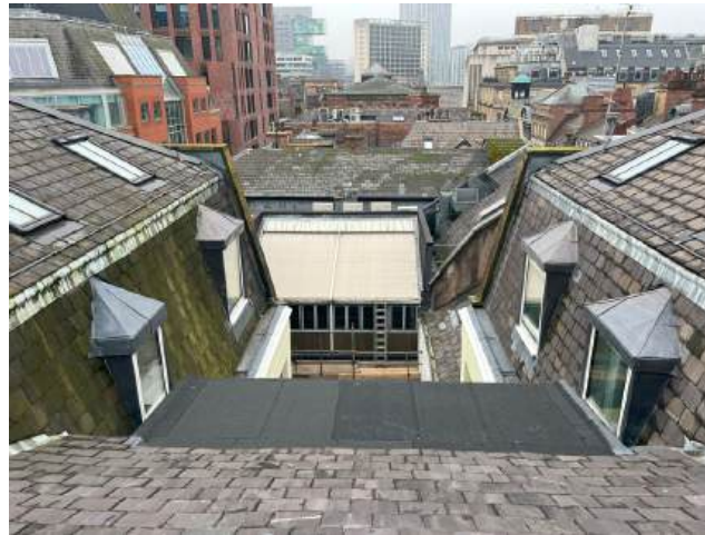
2.13 View of 58-60 King Street from roof of 62 King Street.heic
