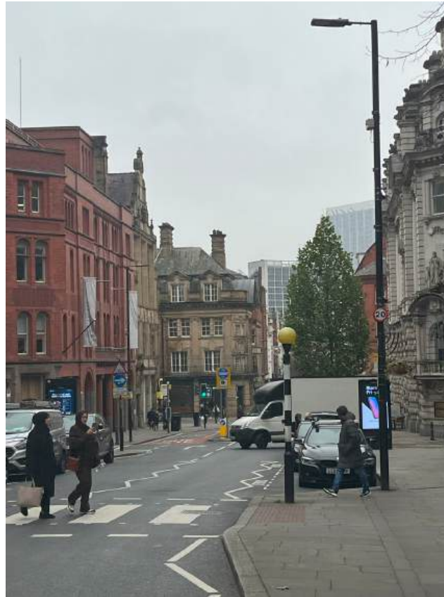
2.5 Apex of 62 King Street gable from East end of King Street beyond Cross Street.heic
