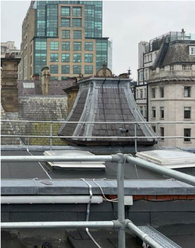
2.22 Concave Mansard roof to 64-66 King Street
