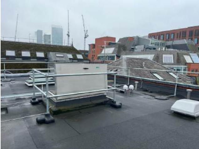
2.18 Substantial plant enclosure looking South-west.heic
