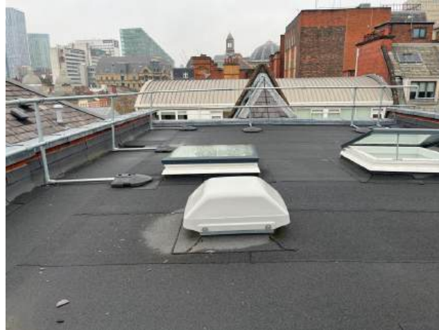
2.20 Pitched roof of gable on 62 King Street facade.heic
