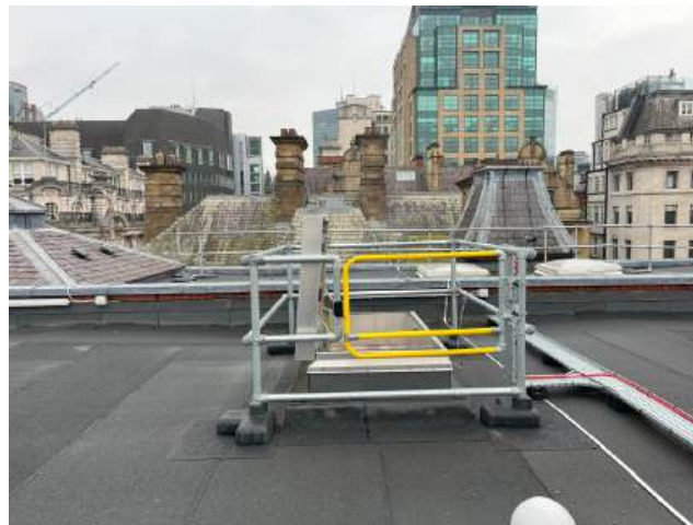
2.14 Access hatch through 62 King Street roofing.heic
