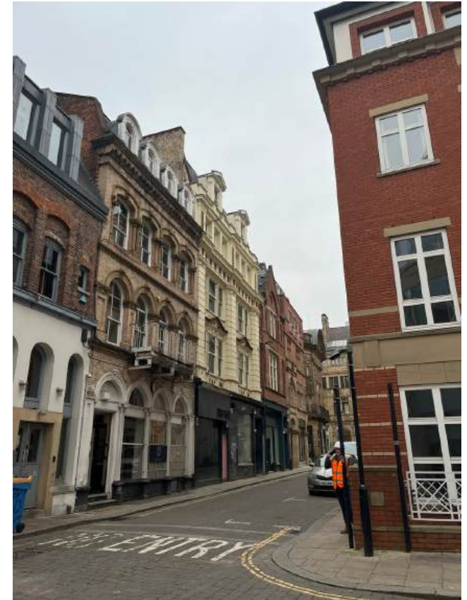
2.6 Built form along South King Street looking East.heic
