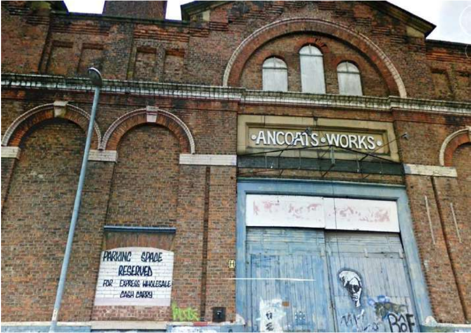
Ancoats Works Pollard Street, Holt Town
