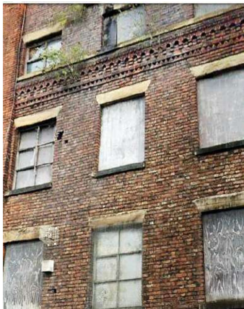
9. Brunswick Mill, Bradford Road, Holt Town- simple , repeated fenestration and brick detailing at key junctions/ locations
