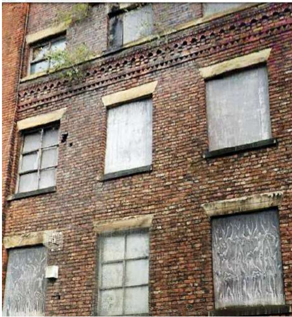
Brunswick Mill, Bradford Road, Holt Town
