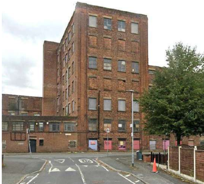
9. Brunswick Mill, Bradford Road, Holt Town
