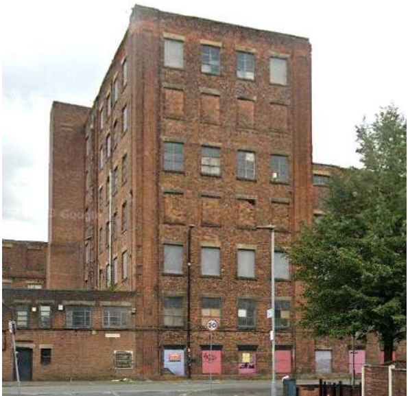
Brunswick Mill, Bradford Road, Holt Town
