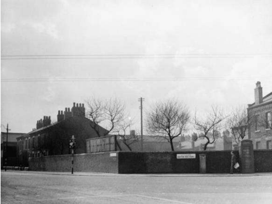
Junction of Grey Mare Lane with Ashton New Road (1962)
