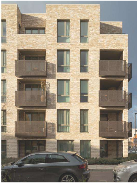
Apartments, London – Macreanor Lavington Architects
