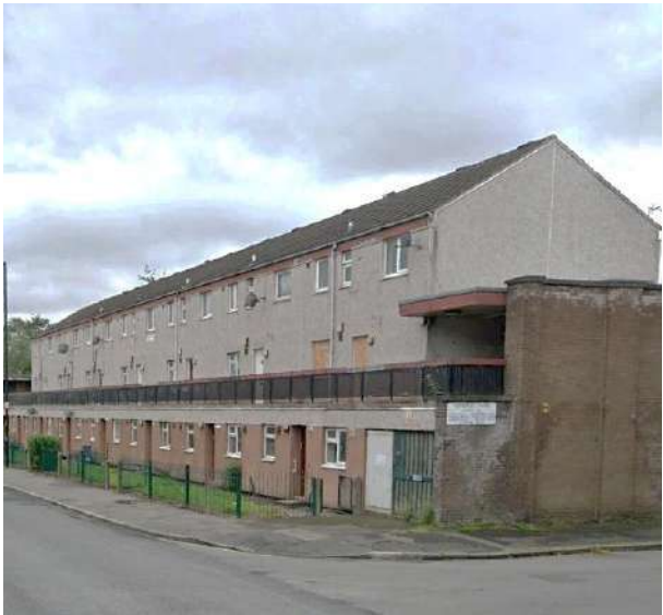
3. 3 storey maisonette flats along Grey Mare Lane
