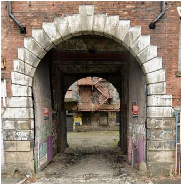
9. Brunswick Mill, Bradford Road, Holt Town- entrance detail
