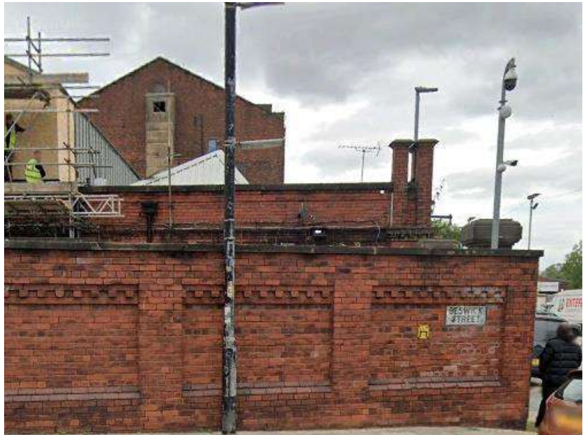
10. Brick detailing, Beswick street, Holt Town/ Ancoats
