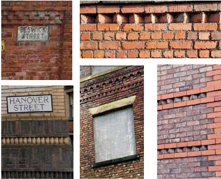
Contextual historic brick detailing
