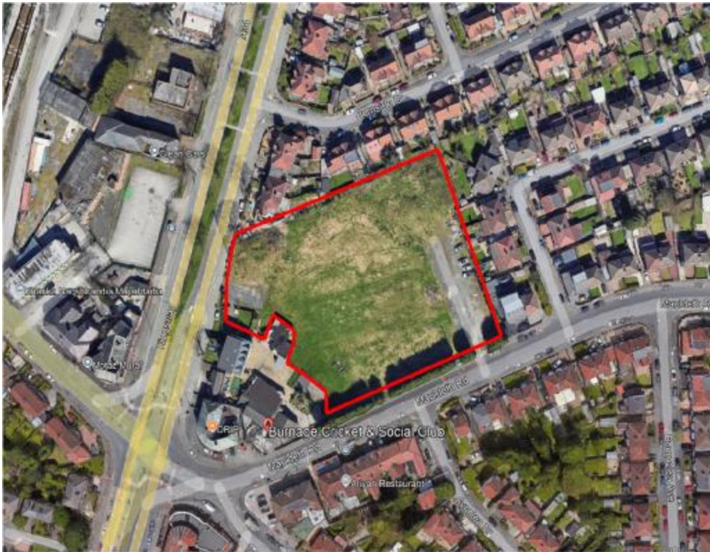
Figure 2 Aerial image of the Burnage Cricket Club site – area to be developed
