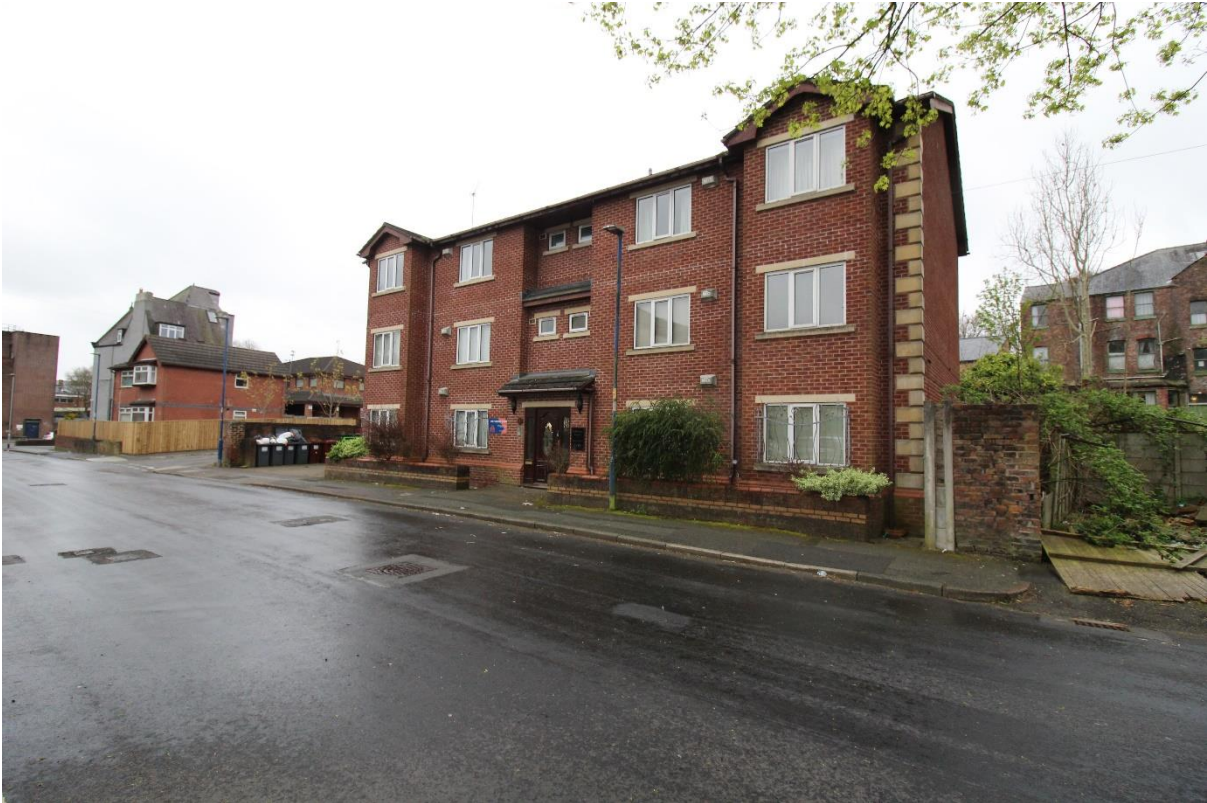
Plate 8 – 1 to 6 Catherine Road to rear of site
