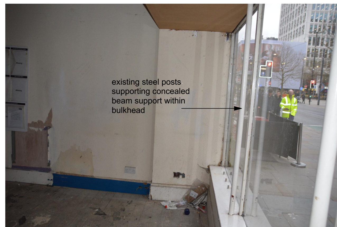
Existing Internal View to Shop Front
