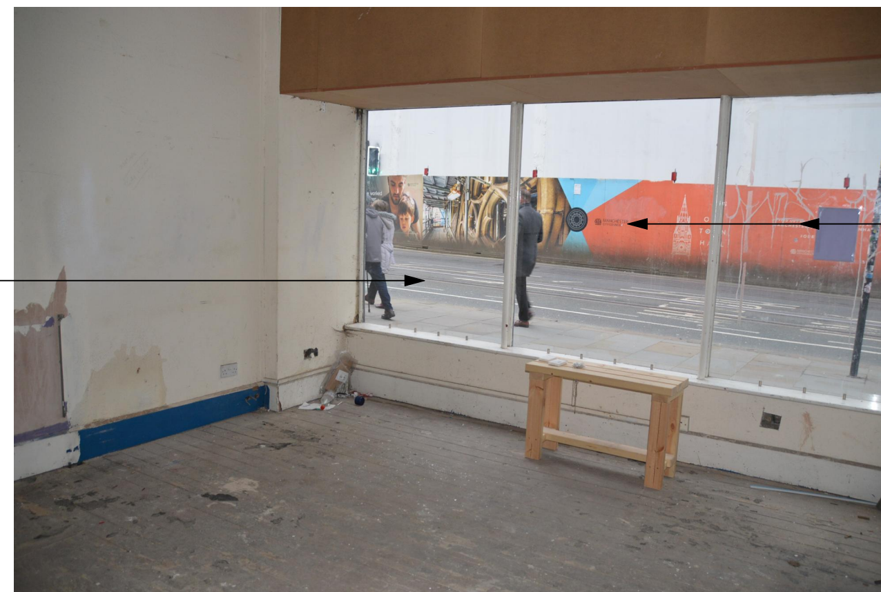
Existing Internal View to Shop Front
