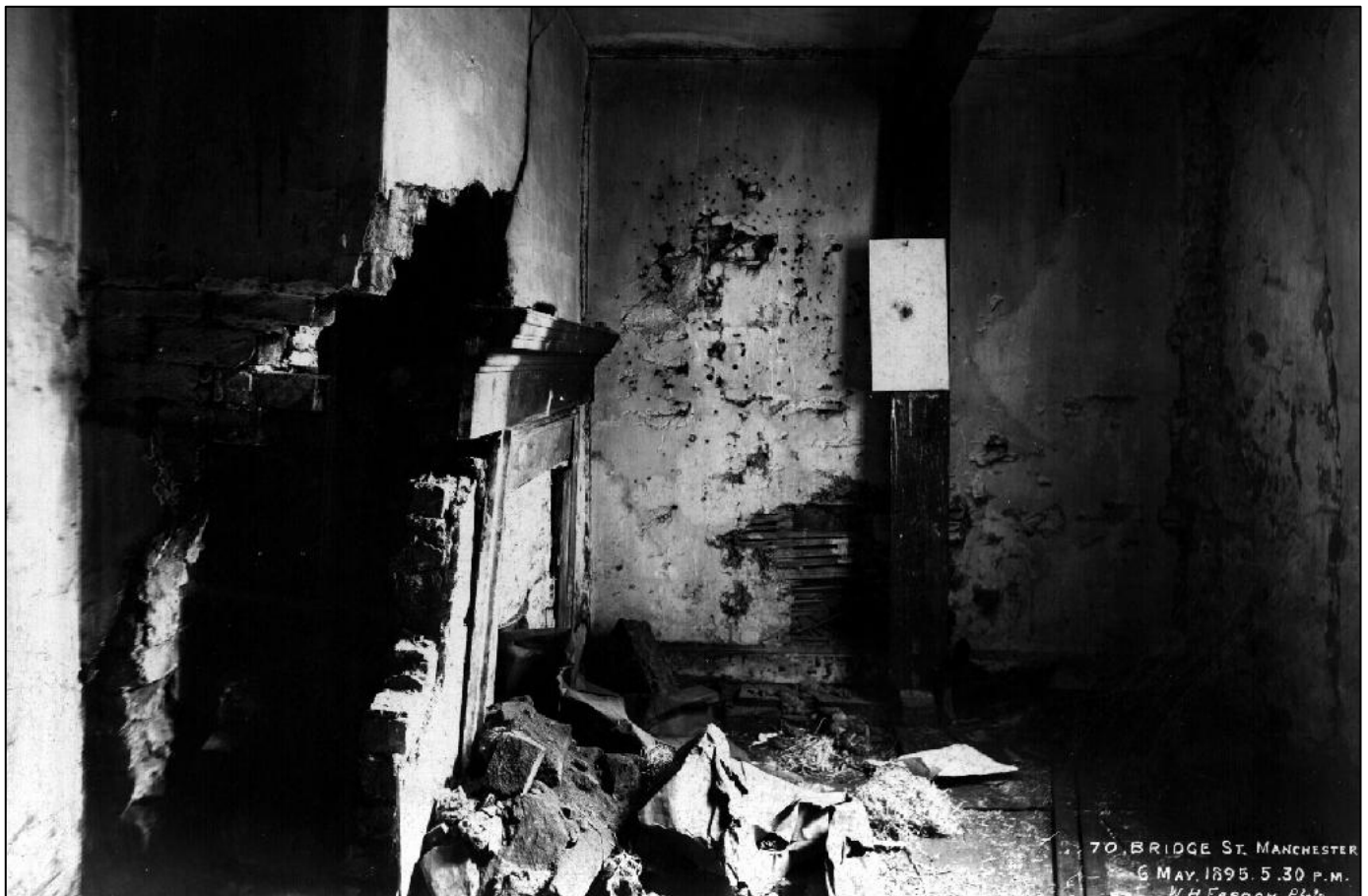
Plate 13 Interior of no. 70 Bridge Street, Manchester, taken in 1895, courtesy of Manchester Local Image Collection
