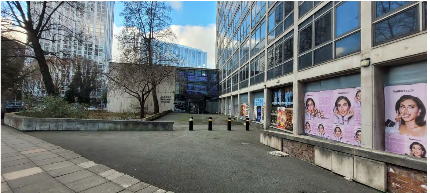
Plate 24 Three-storey entrance building to the west of the main building, looking north-west
