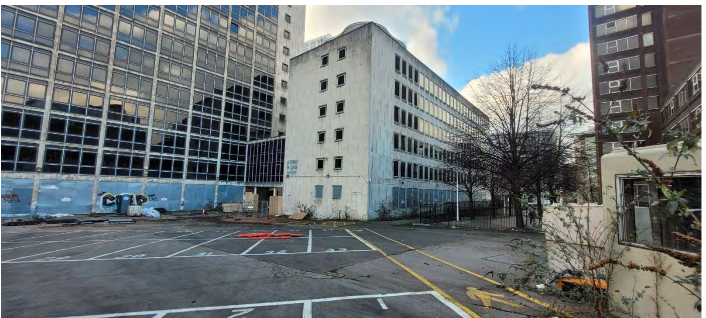
Plate 22 Six-storey building connected to the main tower block, looking north-west
